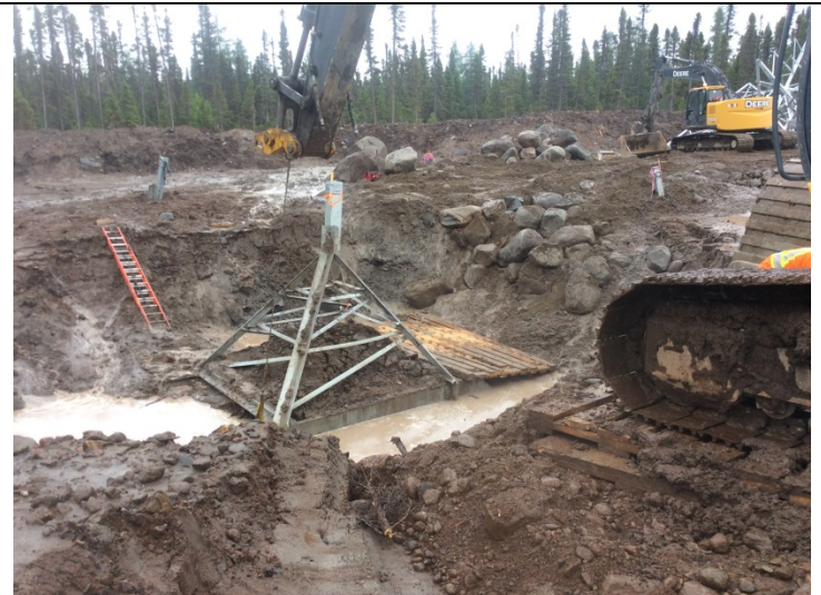
Photo 6: S1-70 Leg A, reclamation of grillage footing.
