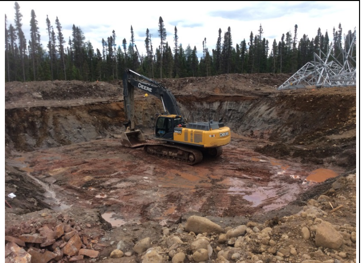
Photo 8: S1-70, common excavation, confirmed weathered bedrock below founding depth.
