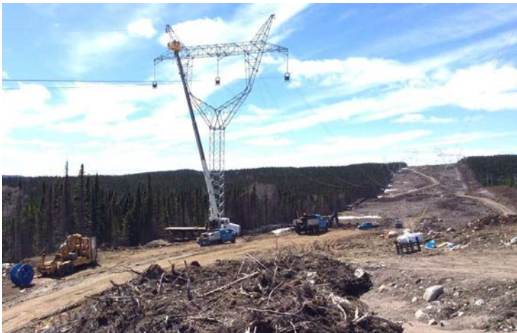
LTA Stringing Operations
