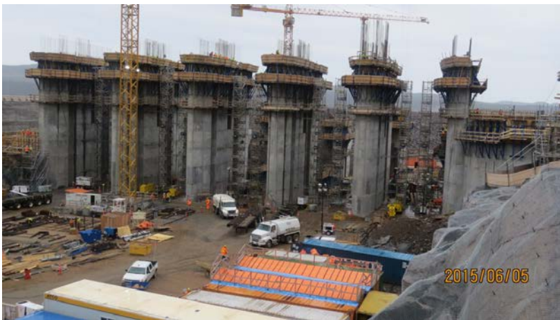
Progress on the Spillway, June 5, 2015
