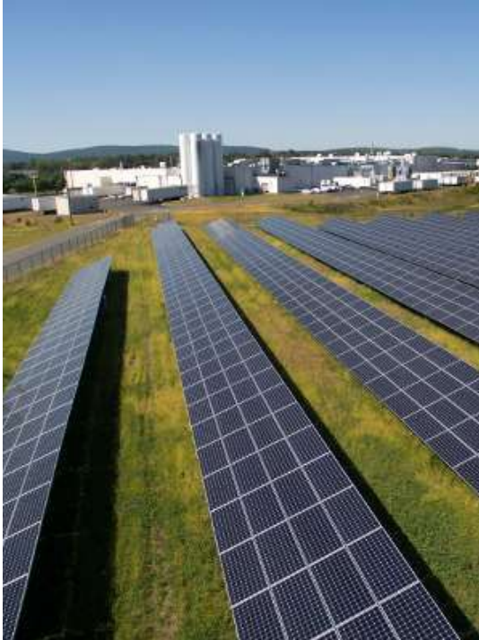
Figure 3: Four-panel high landscape arrangement (courtesy businessfeed.sunpower.com)
