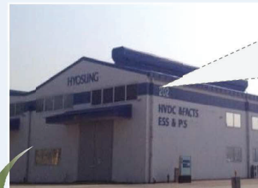
PCS manufacturing factory
