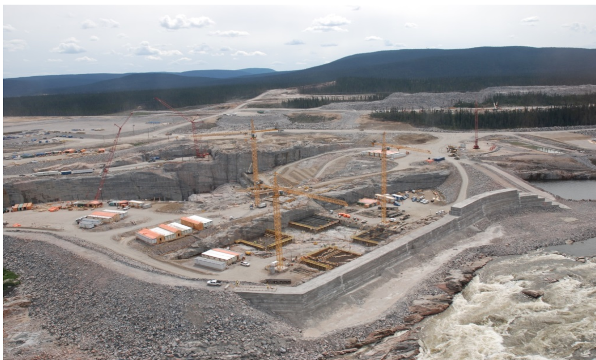
Figure 10-7 – Completion of Bulk Excavation (Powerhouse and Spillway) (shows early construction activity by main civil contractor)
