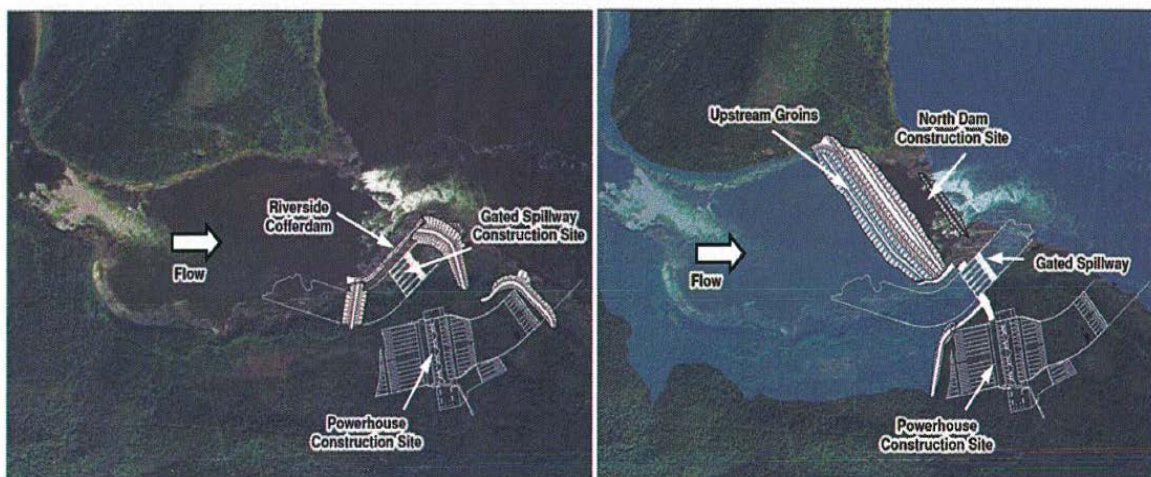
Figure 10-11 – Stage 1 (Pre-Diversion) and Stage 2 (Post Diversion)
