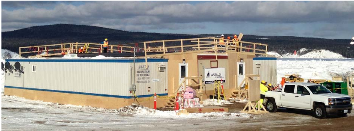
Figure 28: Powerhouse Office Complex – February 2014
