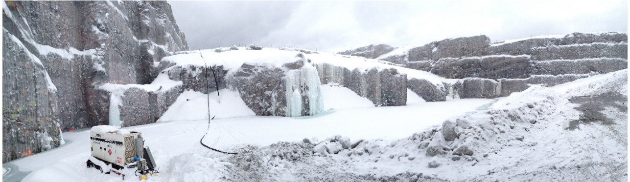
Figure 8: Powerhouse floor – December 2013
