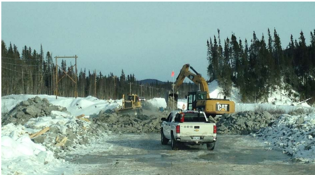
Figure 29: Works at Mackenzie Brook – February 2014
