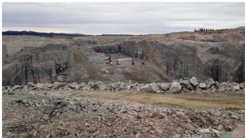
Figure 6: Intake and Powerhouse, downstream view – November 2013
