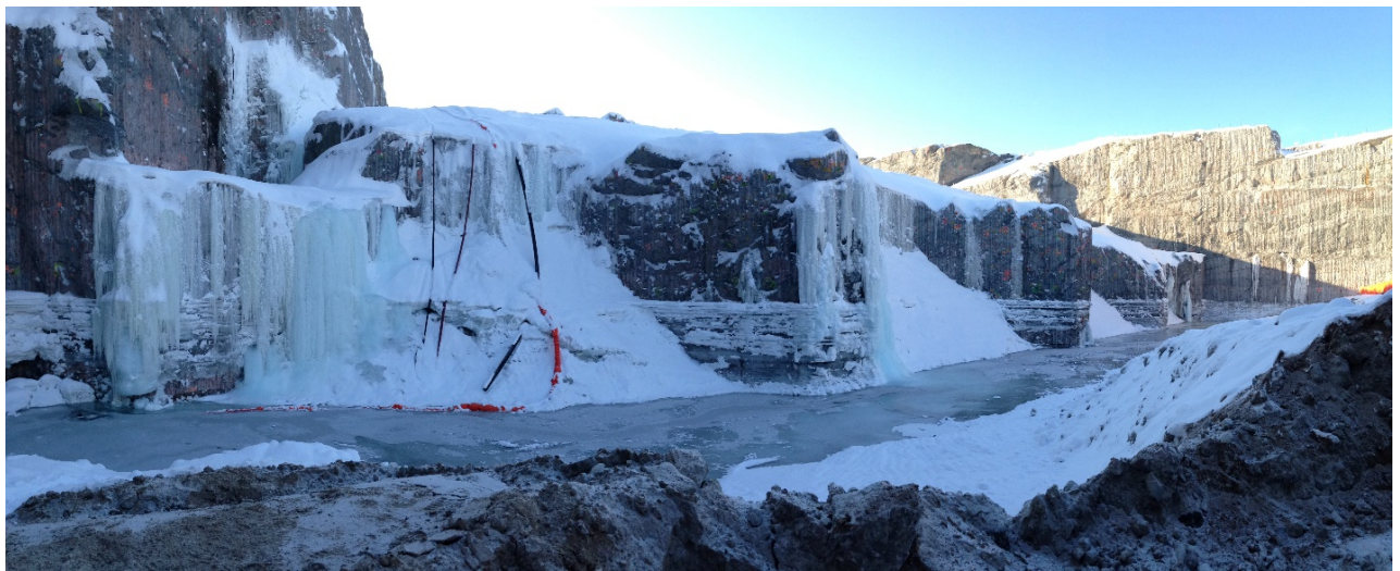
Figure 9: Powerhouse floor – February 2014 – dewatering in progress
