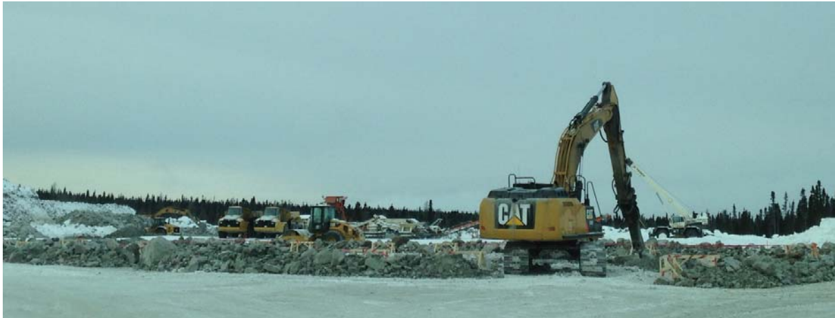
Figure 17: Batching Plant Foundations – January 2014
