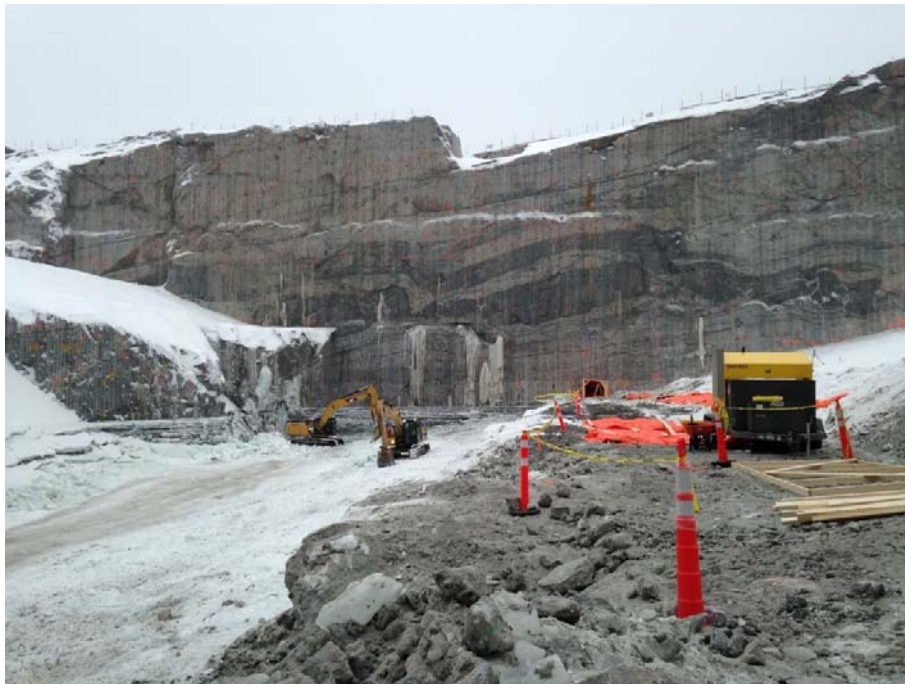
Figure 10: Powerhouse D-Line - rock cleaning – January 2014
