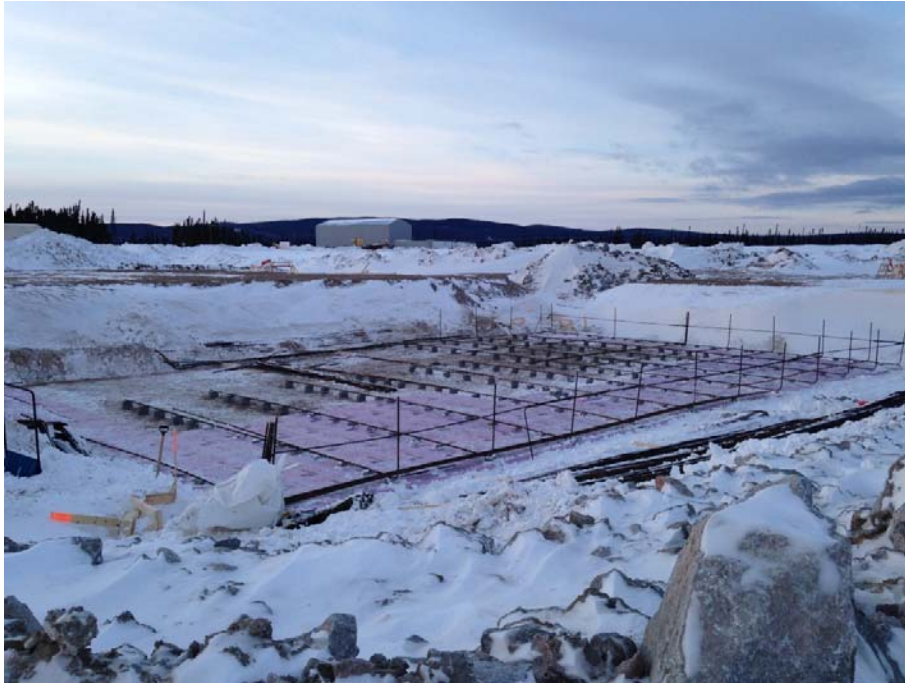
Figure 19: Batching Plant Foundations – February 2014
