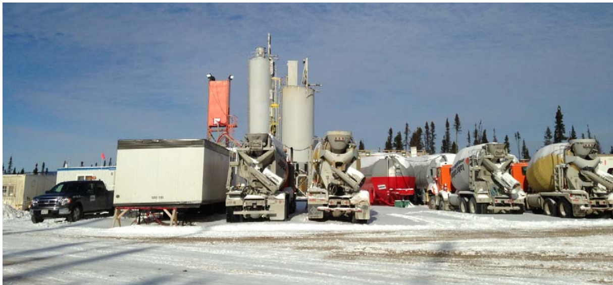
Figure 27: Temporary Batching plant – February 2014
