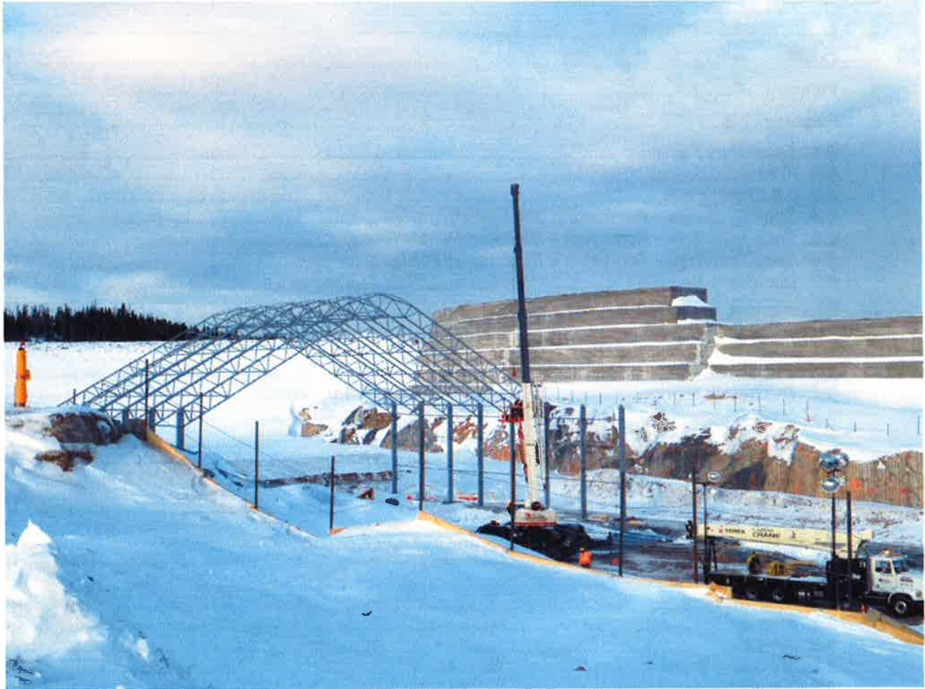
Figure 1: Spillway Cover - 21 February 2014
