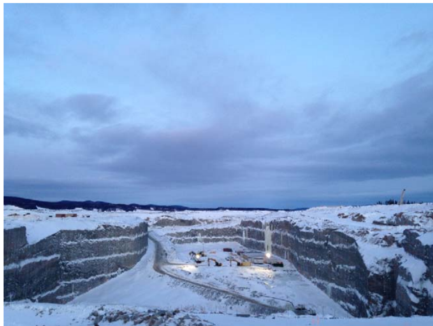
Figure 7: Intake and Powerhouse, downstream view – February 2014
