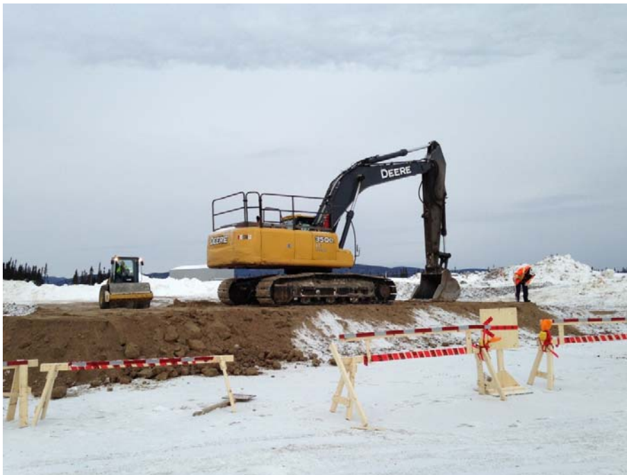
Figure 18: Batching Plant Foundations – February 2014
