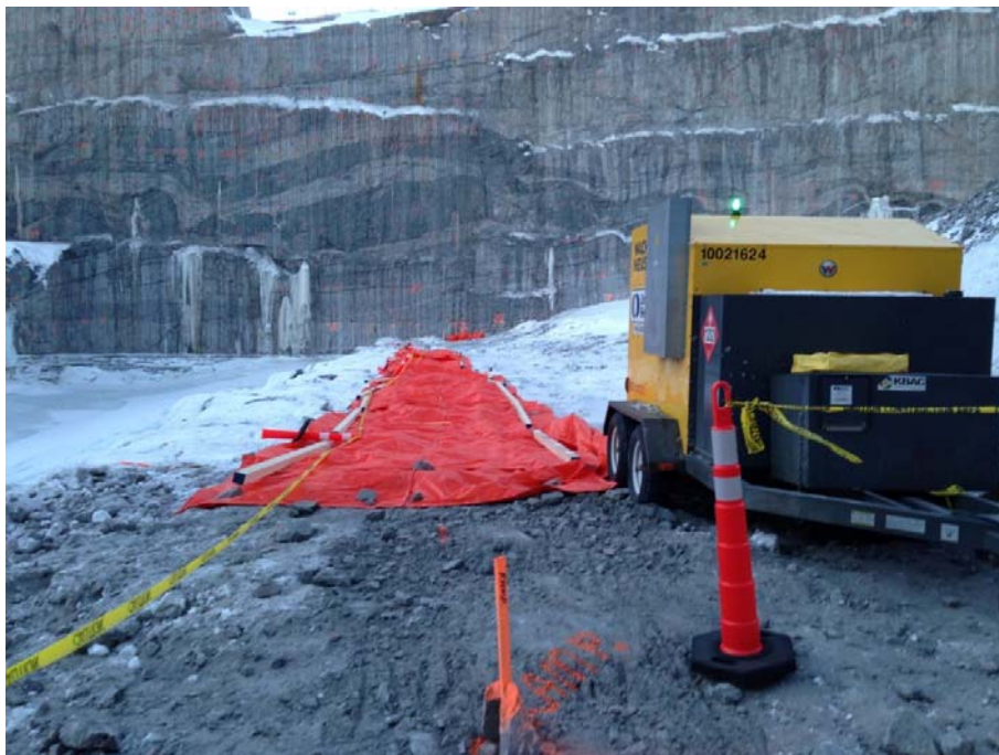
Figure 11: Powerhouse D-Line – rock cleaning – January 2014
