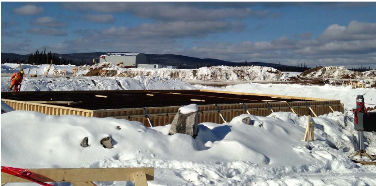
Figure 20: Batching Plant Foundations – February 2014
