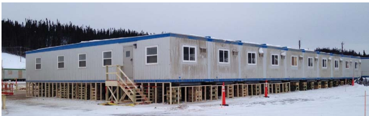
Figure 32: Laydown Area – Main Office Complex - February 2014
