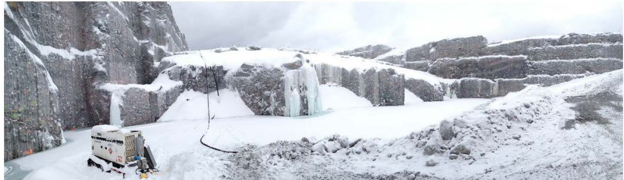
Figure 8: Powerhouse floor – December 2013
