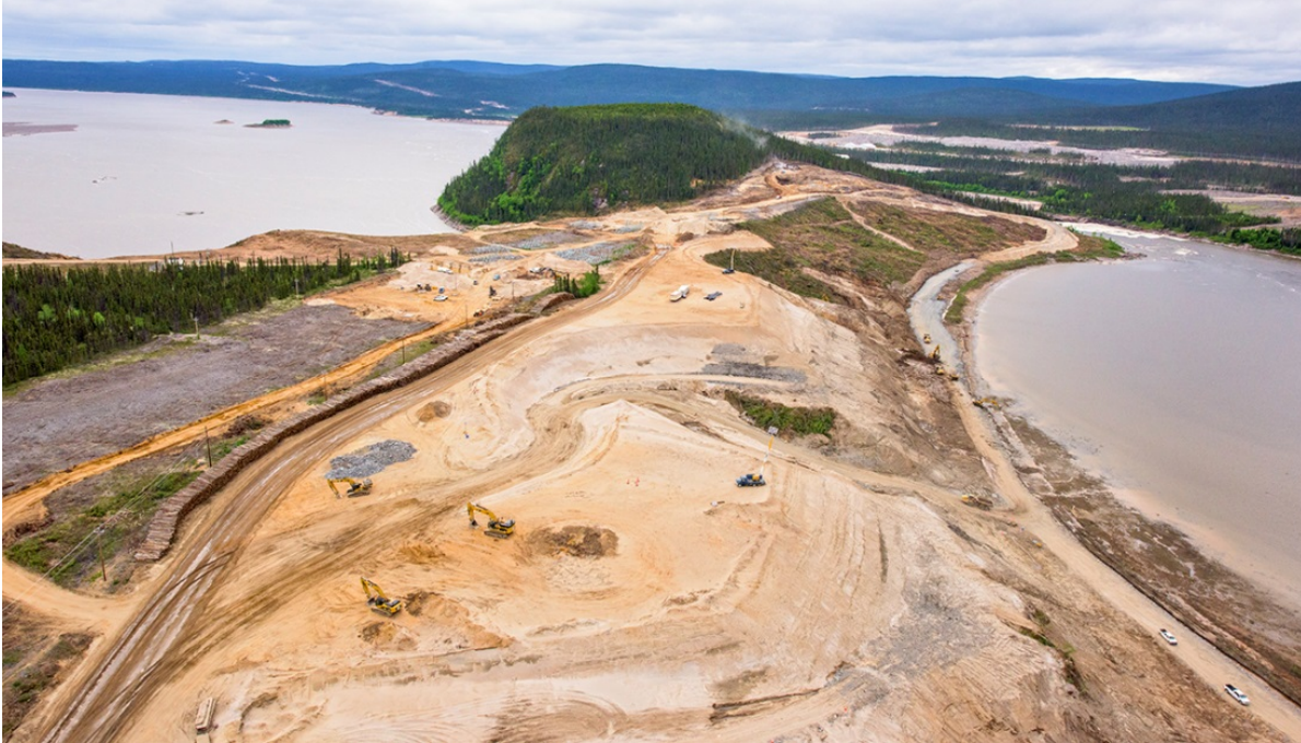
Muskrat Falls Site – Progress on North Spur – August 2015
