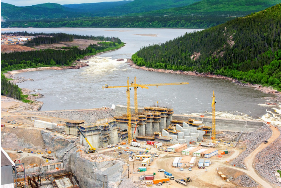
Muskrat Falls Site – Progress on Spillway and Powerhouse – August 2015
