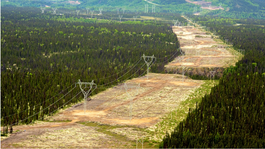
Progress on the HVac Transmission Line (Labrador Transmission Assets) – August 2015
