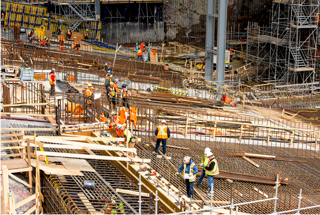
Progress on the Powerhouse at the Muskrat Falls Site – August 2015
