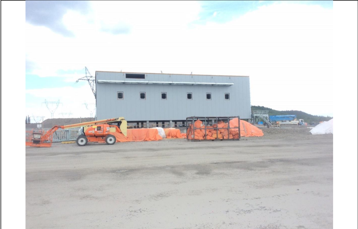
Photo H.5: Exterior view of fully erected GIS Building. (July 14, 2016)
