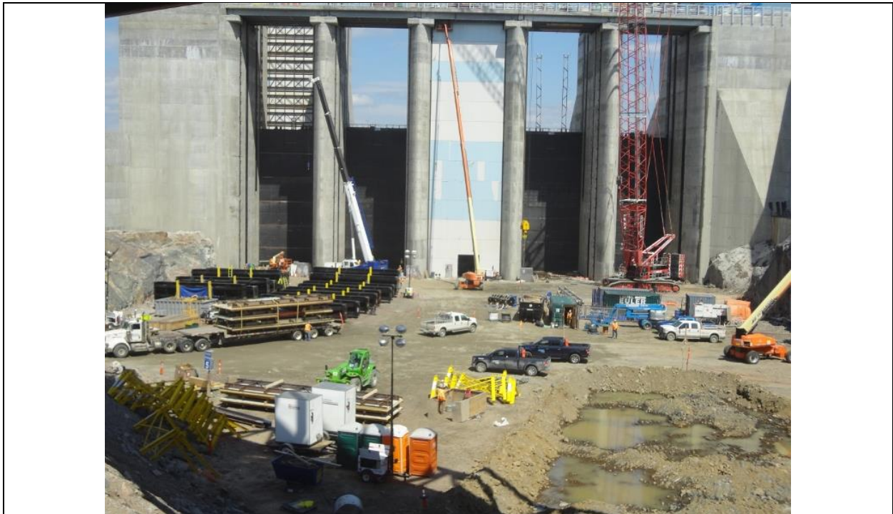
Photo D.2: Upstream view of the spillway gates. (July 13, 2016)
