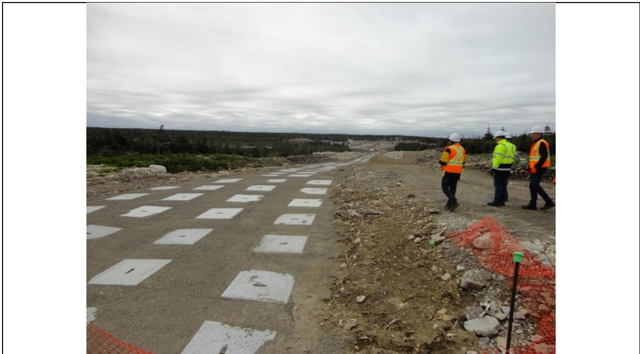
Photo A.8: View looking eastwards along the buried cables line. (July 12, 2016)
