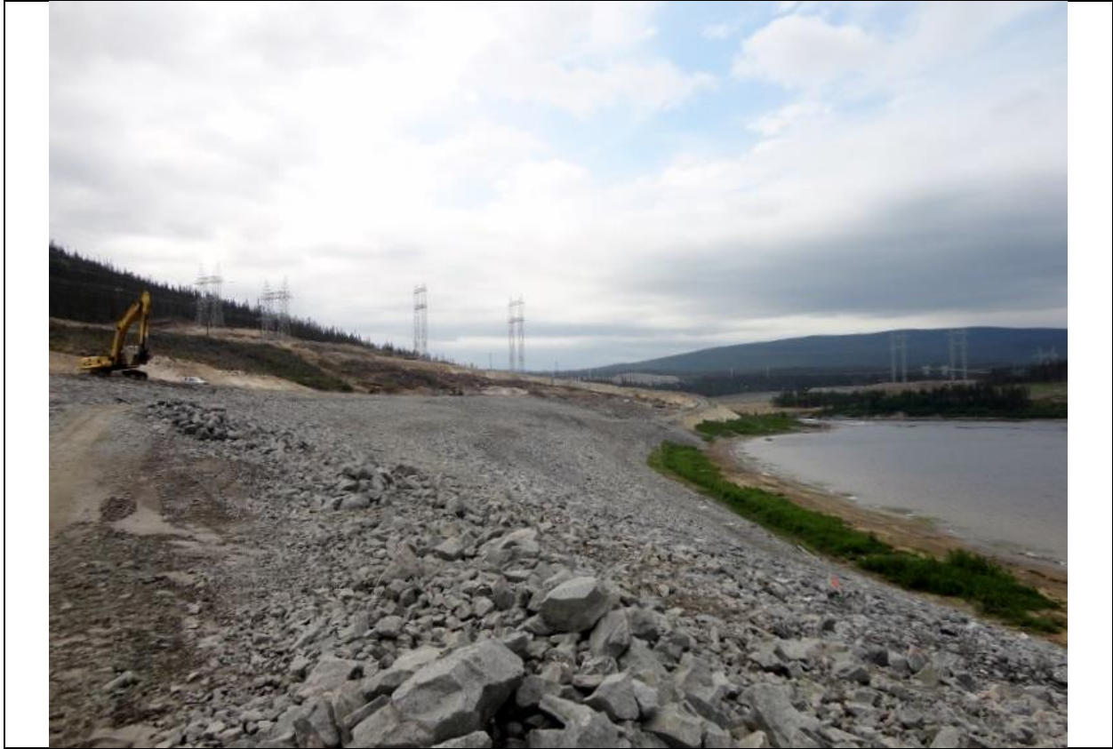
Photo E.3: North Spur, upstream slope. View looking south. (July 14, 2016)
