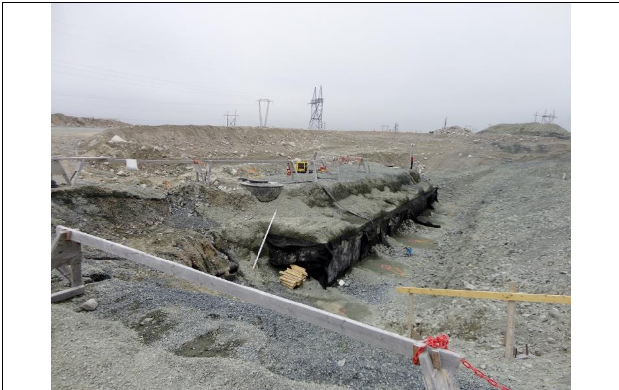
Photo I.8: Soldiers Pond – Converter Station oil / water separator tank partially backfield. (July 15, 2016)
