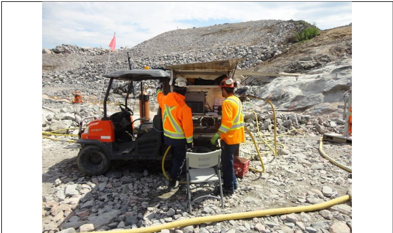
Photo F.6: Grout monitoring station at the South Dam foundation. (July 14, 2016)
