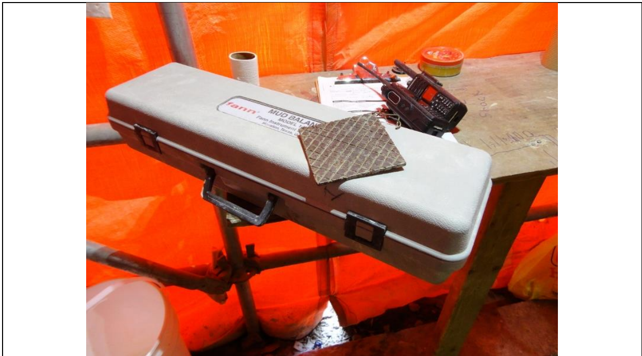
Photo F.10: Spillway grouting gallery, Lombardi type grout cohesion measuring plate for use with GIN grouting. (July 14, 2016)
