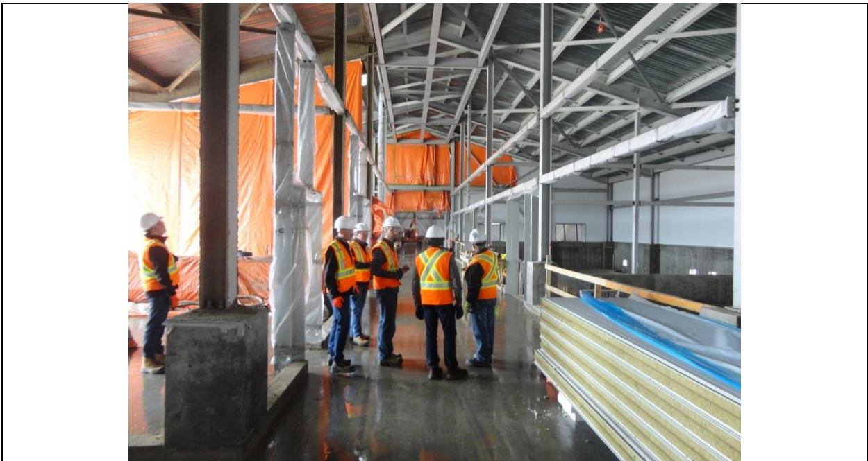
Photo I.2: Soldiers Pond – Converter Station control room interior. (July 15, 2016)
