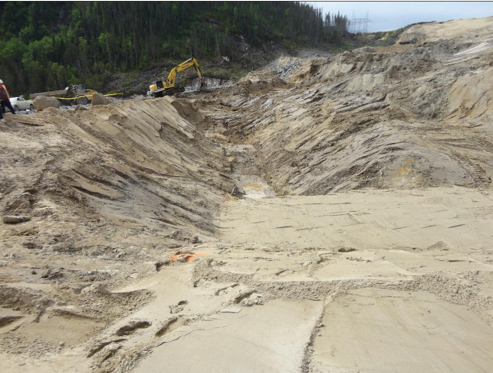
Photo E.12: North Spur, downstream slope. Sloping finger drain. (July 14, 2016)
