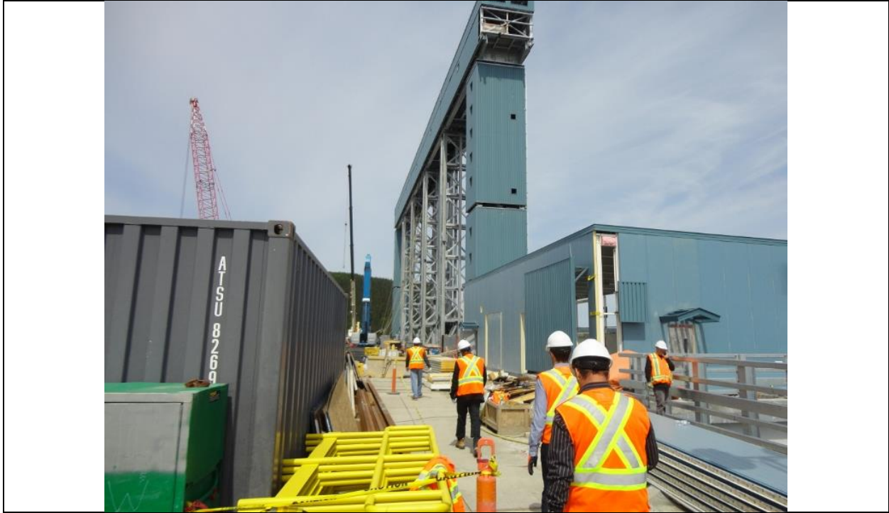
Photo D.5: Deck on top of the spillway gate structure. (July 13, 2016)
