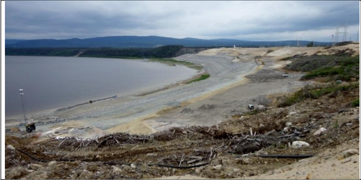
Photo E.1: North Spur, upstream slope. (July 14, 2016)
