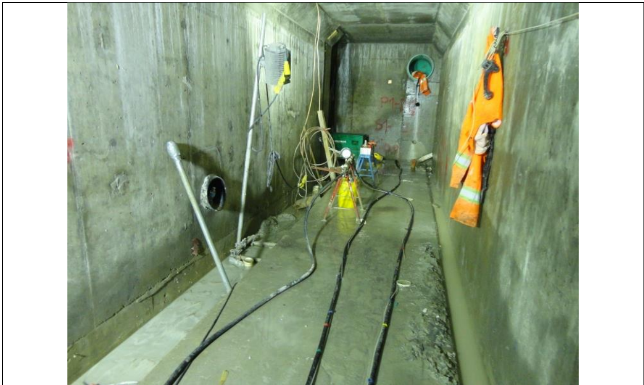
Photo F.8: Powerhouse Intake grouting gallery, south end. (July 14, 2016)
