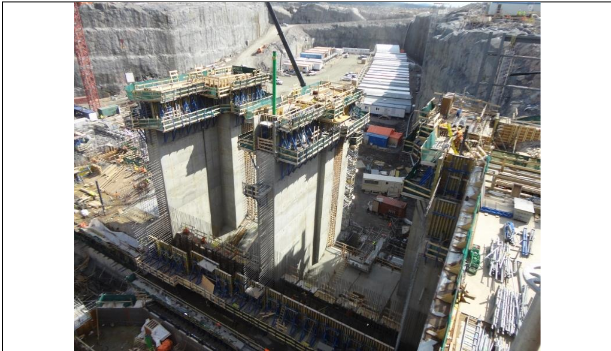
Photo C.6: Concrete walls at intake of Unit 1, view looking downstream. (July 13, 2016)
