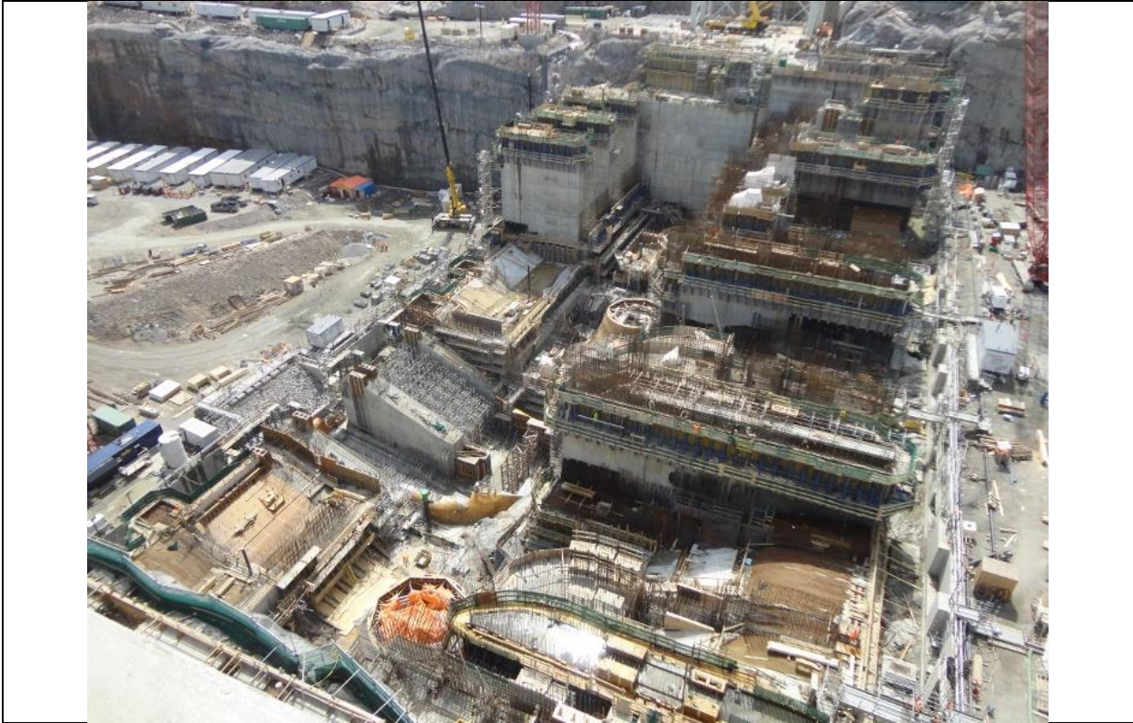
Photo C.3: View of powerhouse from spillway area looking south. (July 13, 2016)
