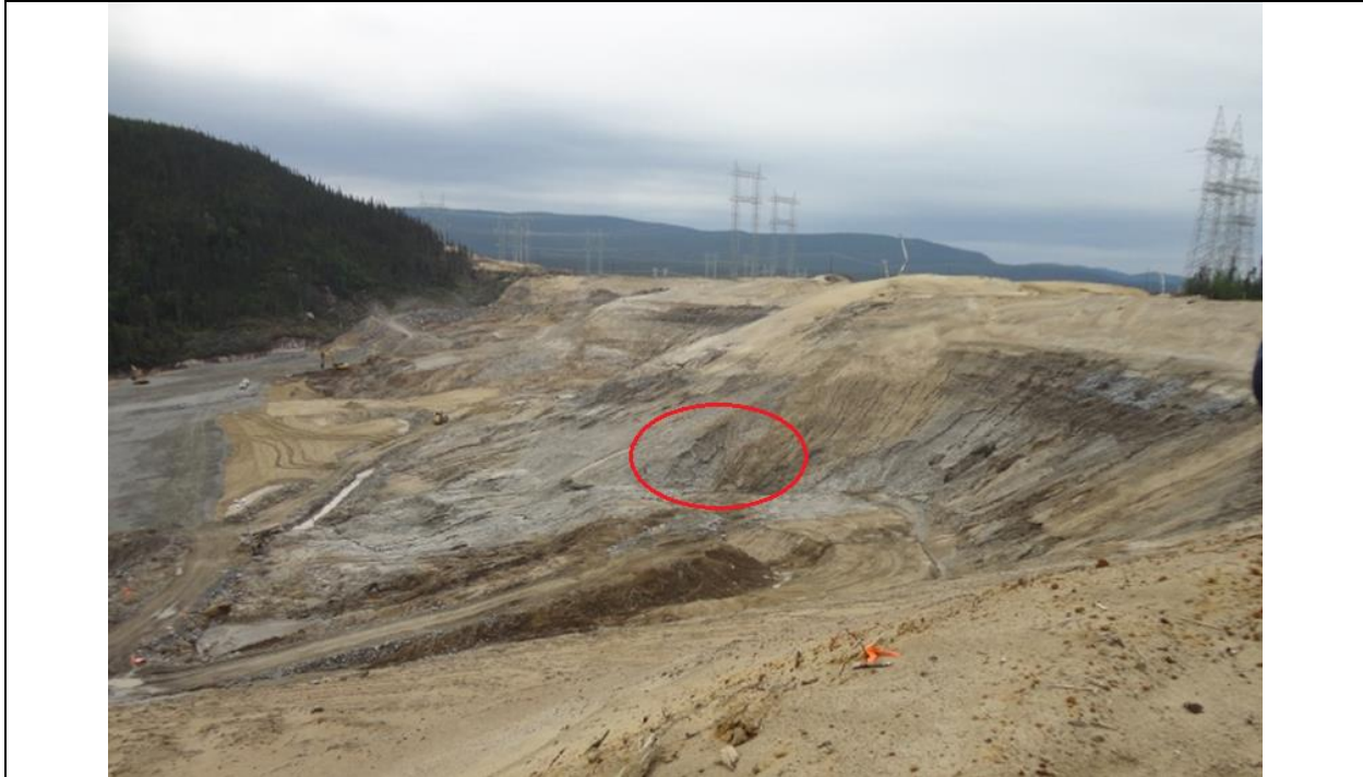
Photo E.9: North Spur, upper level of the downstream slope. Area where liquefiable material was encountered in 2015 is outlined by the red ellipse. (July 14, 2016)
