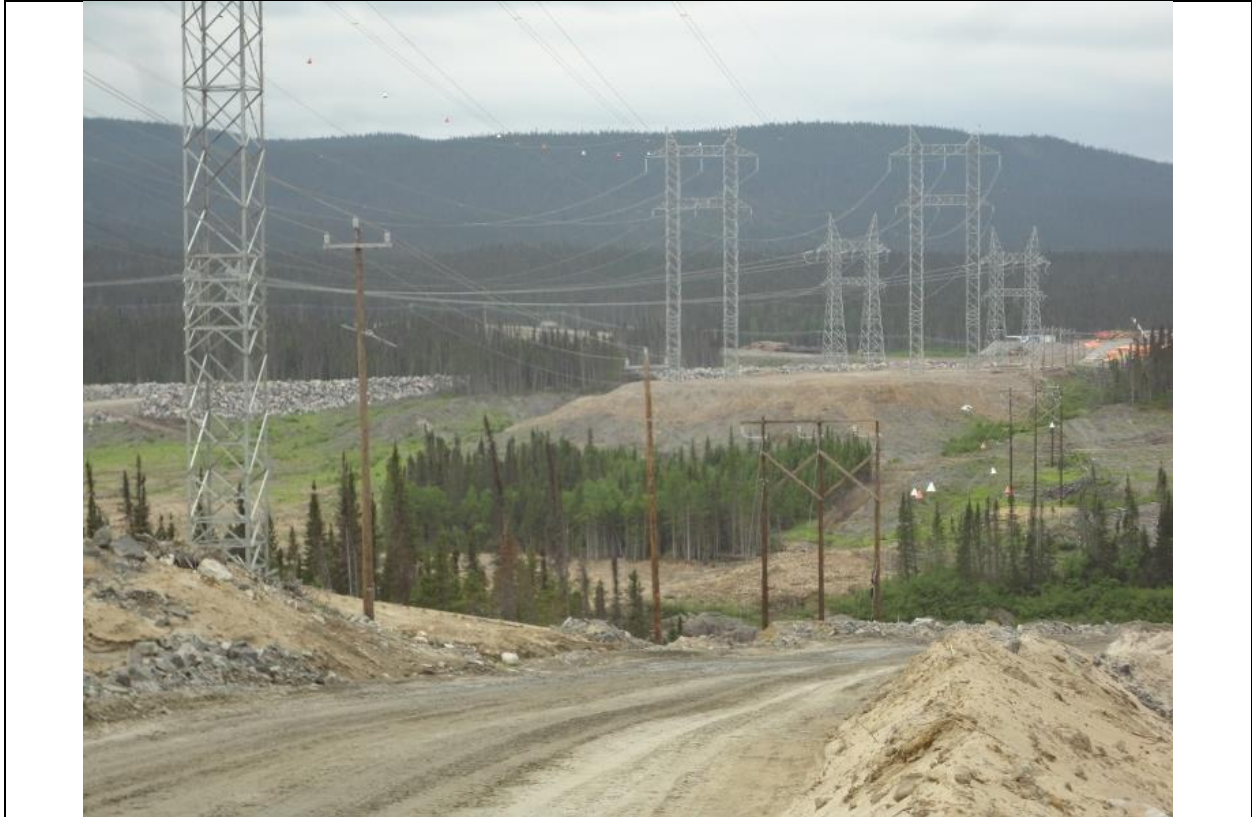
Photo E.7: North Spur. View looking north at the HVac transmission line along the top of the North Spur. (July 14, 2016)
