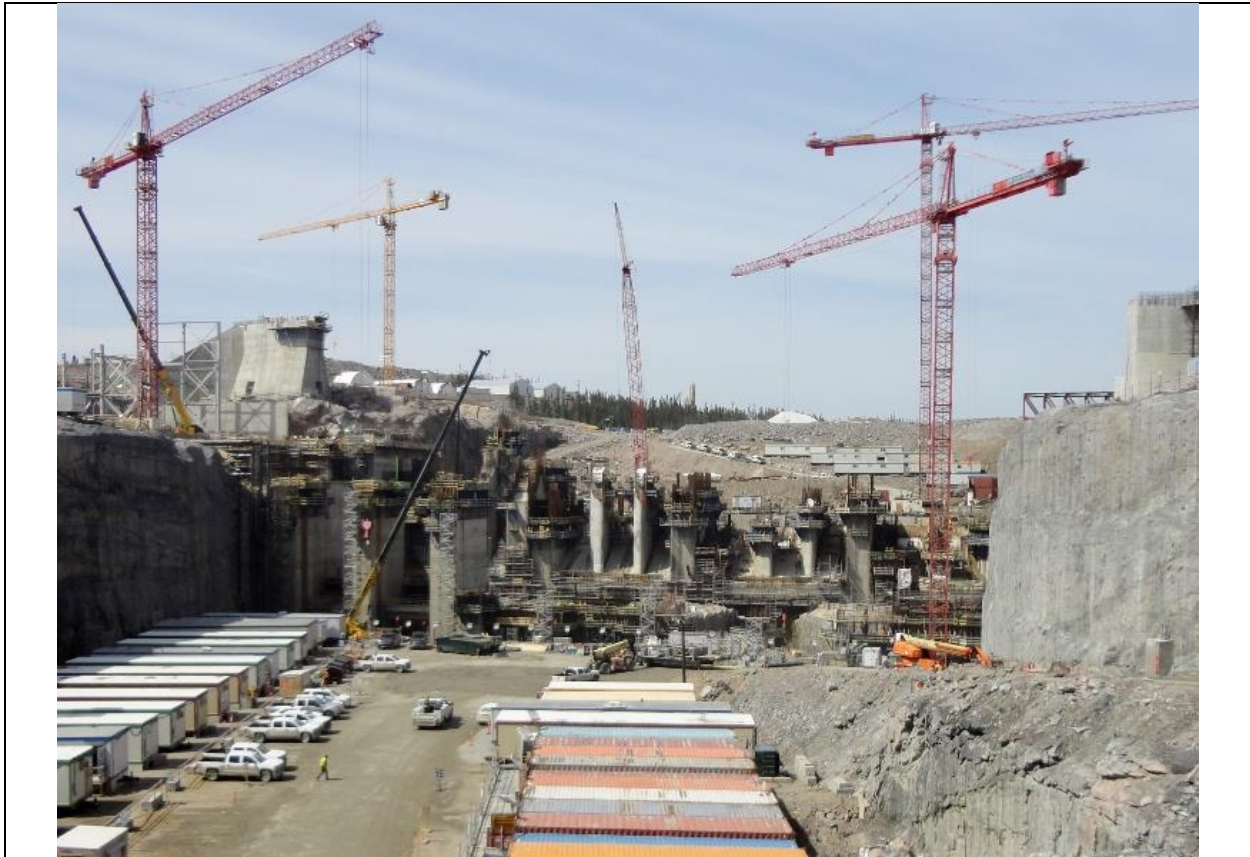
Photo C.1: Downstream face of the powerhouse. (July 13, 2016)
