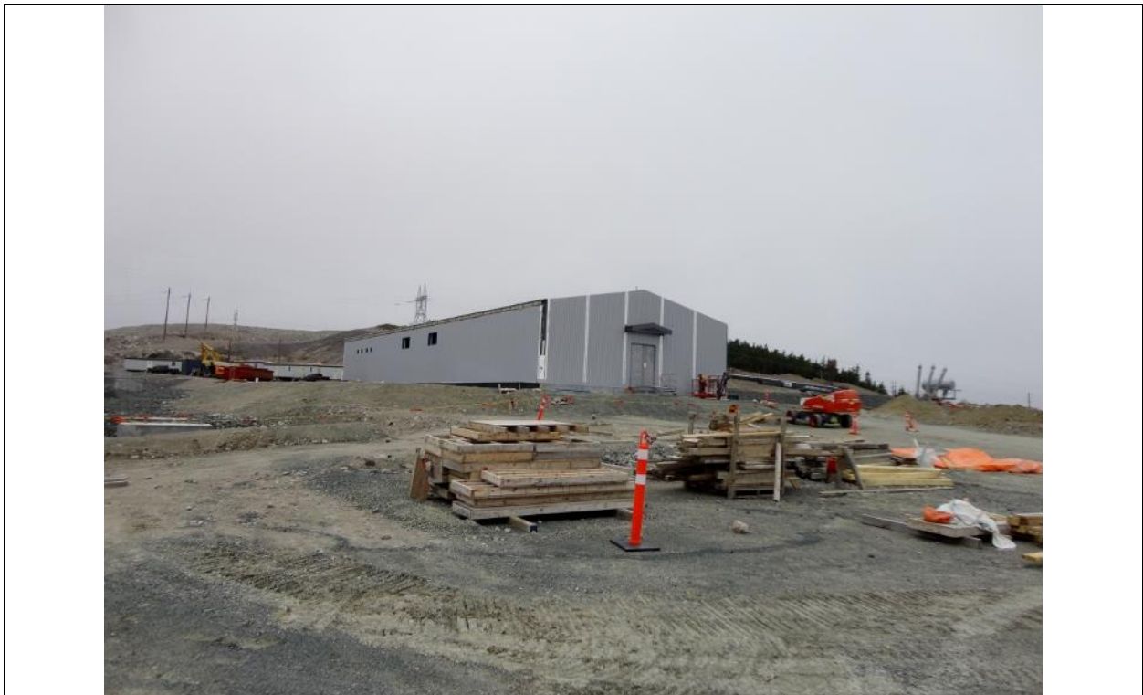
Photo I.10: Soldiers Pond – Control building fully assembled. (July 15, 2016)
