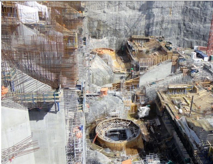
Photo C.10: Units 2, 3 and 4. (July 13, 2016)
