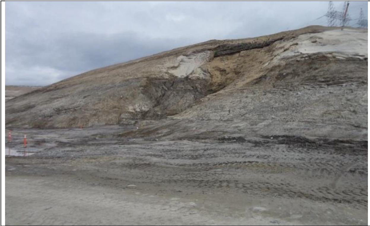
Photo E.5: North Spur, upstream slope. Old gully scar at the mid-point. (July 14, 2016)
