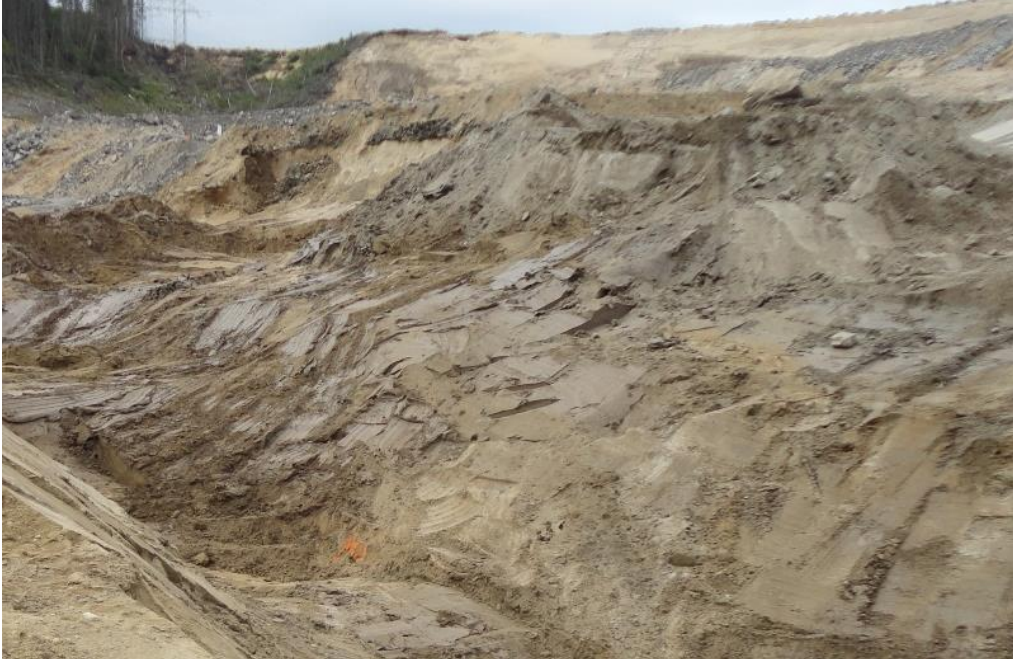
Photo E.11: North Spur, downstream slope. Exposure of plastic silt/clay with interlayered fine sand of the Upper Stratified Drift. This location is near in the southern area at the base of the downstream slope. No evidence of liquefaction properties could be seen at this location. (July 14, 2016)
