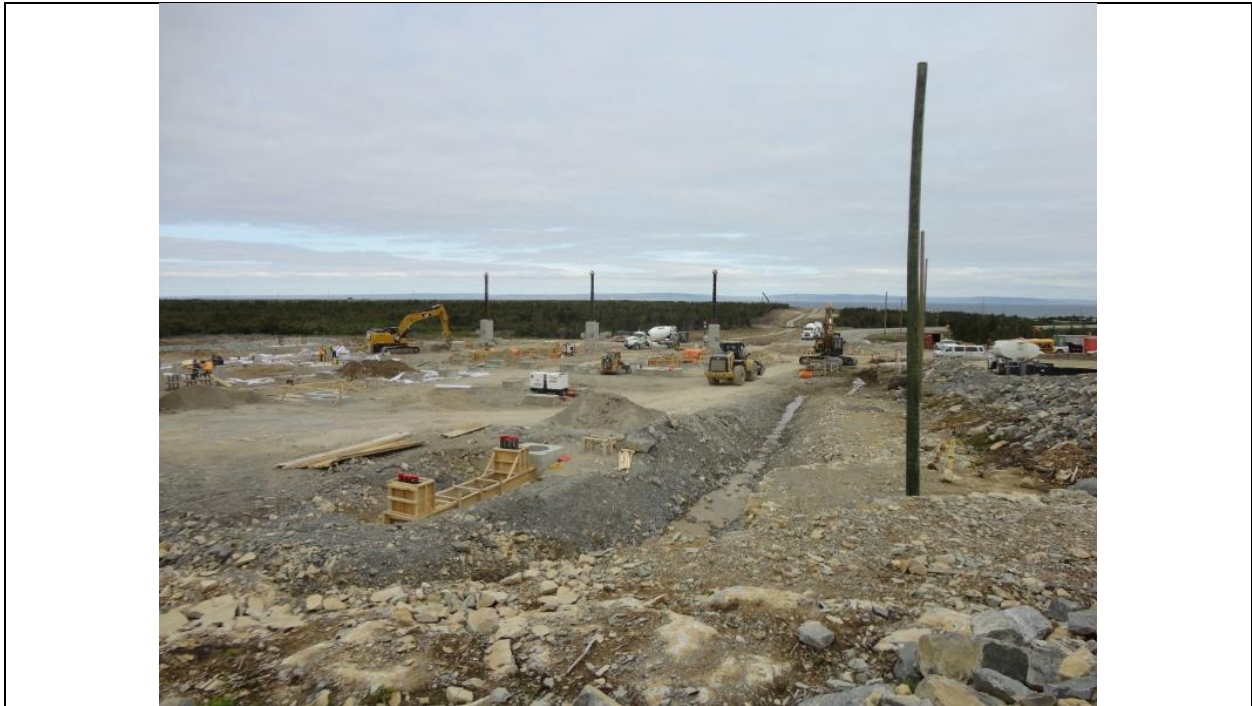
Photo A.10: Shoal Cove Transition compound preparatory works. (July 12, 2016)
