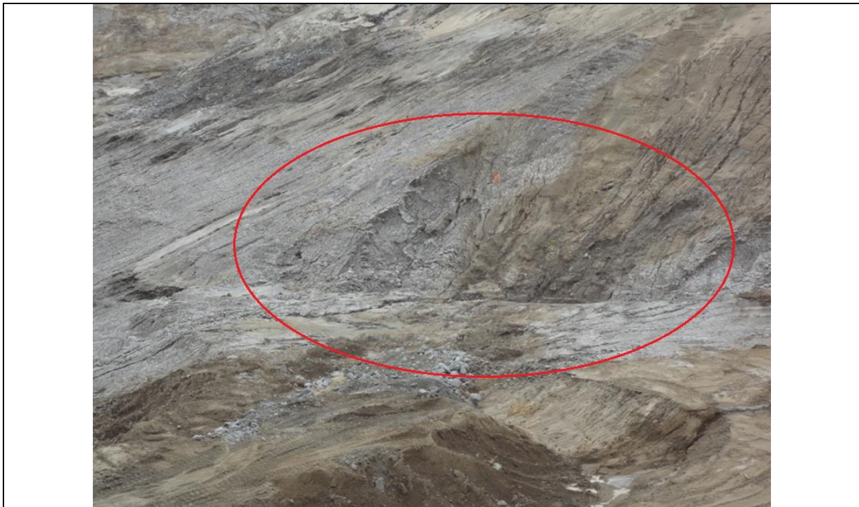
Photo E.10: North Spur, downstream slope. Close-up view of the area where liquefiable silt/clay was reportedly excavated during 2015 (See Photo E.9 above). It was reported that material obtained from this area was liquefied when loaded into dump trucks, it flowed out of the back of the truck as it climbed the slope. To date no further information on the extent or properties of this liquefiable material has been presented to the IE. (July 14, 2016)
