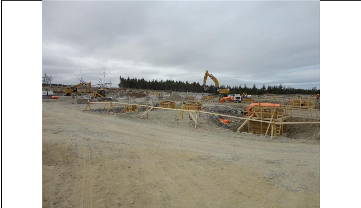
Photo A.11: Shoal Cove Transition compound preparatory works. (July 12, 2016)
