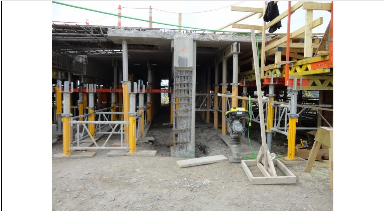
Photo G.5: Close-up of foundation column in stage of repair. (July 13, 2016)
