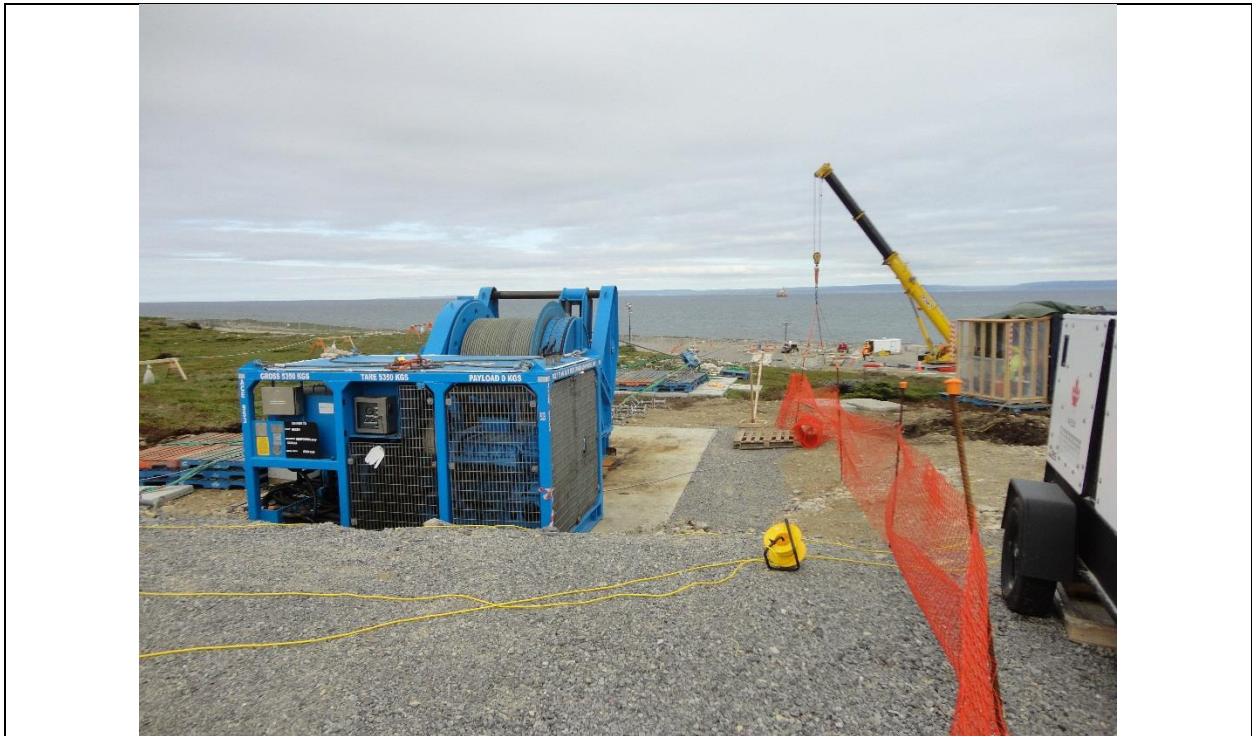
Photo A.6: Winch pulling Cable No 2. (July 12, 2016)
