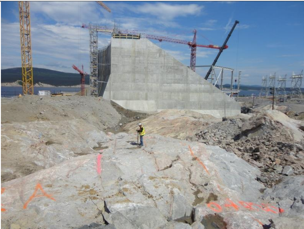
Photo F.4: North end of the South Dam foundation. Cleaned, irregular granitic gneiss in foreground and the south end of the concrete transition dam is in the background. (July 14, 2016)
