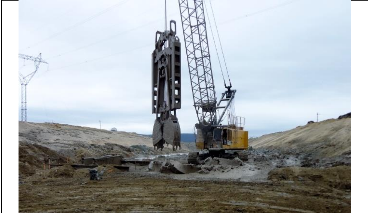
Photo E.15: Dumping of clay material from the North Cutoff. (July 14, 2016)
