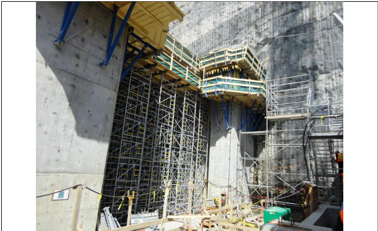
Photo C.8: Intake face for Unit 1. (July 13, 2016)
