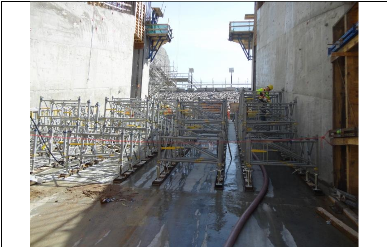
Photo C.15: Unit 3 intake chute, view looking upstream. (July 13, 2016)
