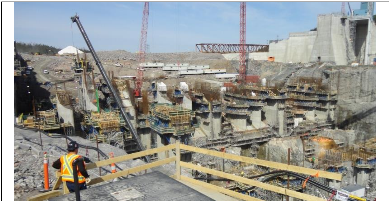
Photo C.2: View of powerhouse looking northwest. (July 13, 2016)
