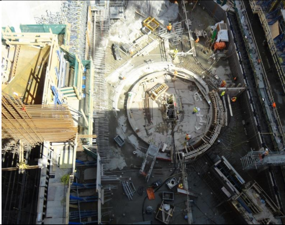
Photo C.9: Unit 1, Draft tube formwork. (July 13, 2016)
