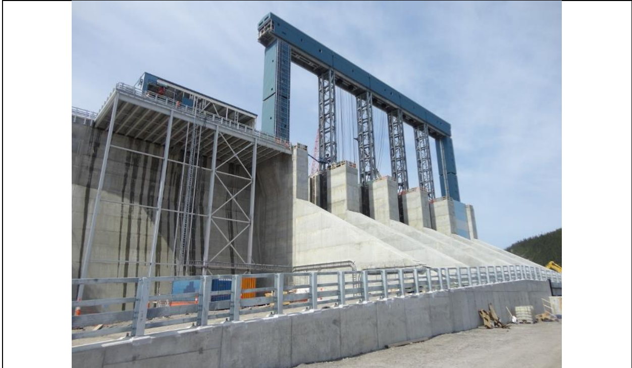
Photo D.1: Downstream view of the spillway gate structure. (July 13, 2016)
