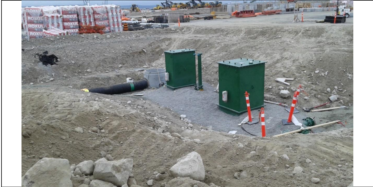
Photo I.17: Soldiers Pond – Synchronous Condenser oil / water separator, partially backfield. (July 15, 2016)
