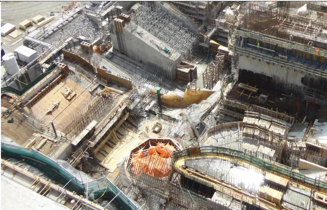
Photo C.13: Units 4 and 3, view looking east; Unit 4 is nearest the camera. (July 13, 2016)
