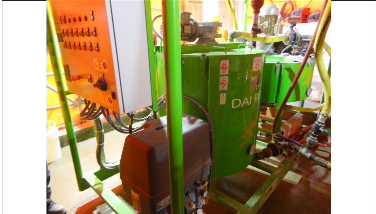
Photo F.11: Spillway grouting gallery, grout mixing plant. (July 14, 2016)
