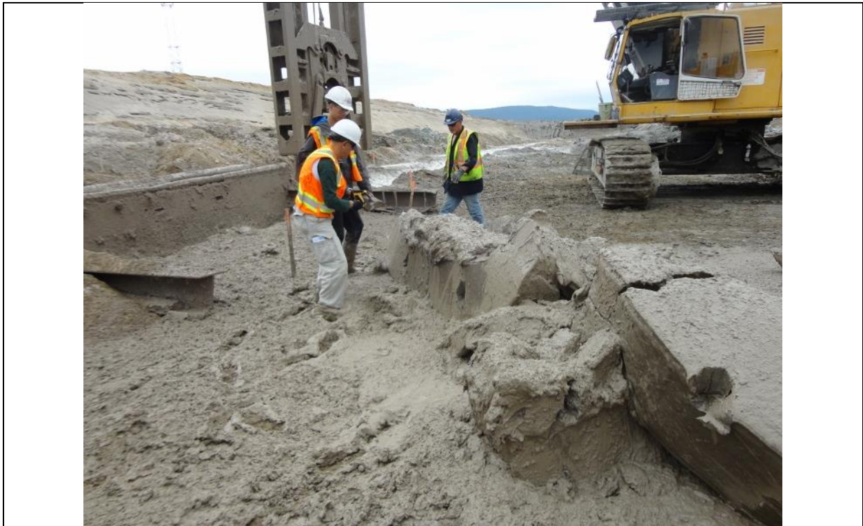
Photo E.16: Plastic "lower clay" from the base of the north Cutoff. (July 14, 2016)
