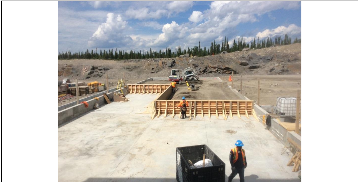
Photo H.7: Concrete foundations of Control Building near completion. (July 14, 2016)
