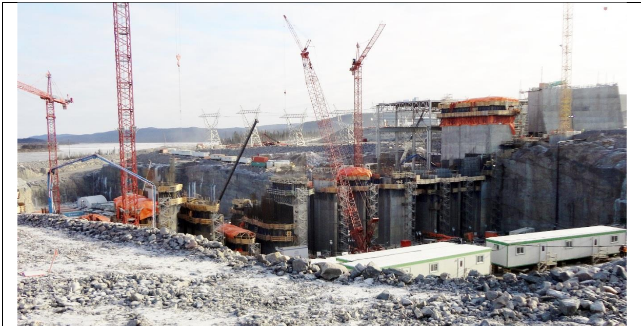
Photo B.4: Looking downstream at the powerhouse intake structures. (November 30, 2016)
