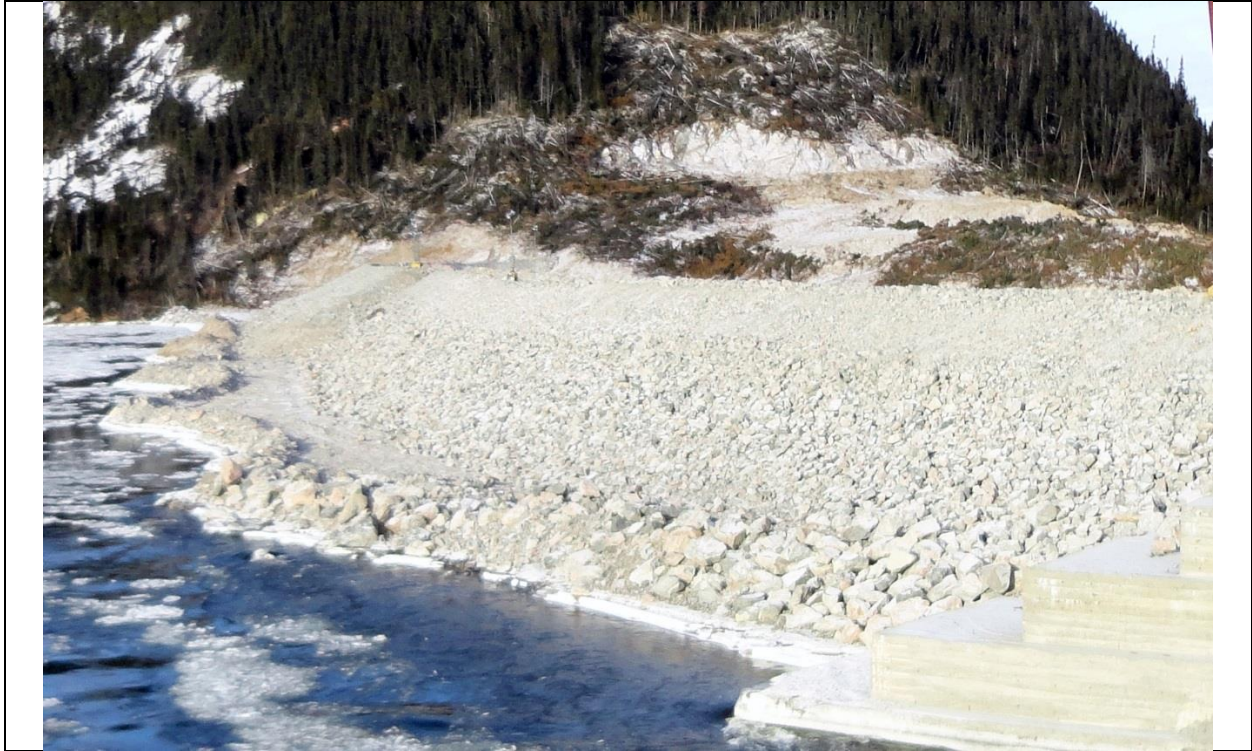
Photo D.9: Upstream face of the cofferdam. The original upstream el 14 m berm is visible along the toe of the dam. The new rockfill paced over the north end of the cofferdam is visible in the far end of the slope. Some new rock fill has also been placed on the upstream slope of below the el 14 m berm. (November 30, 2016)
