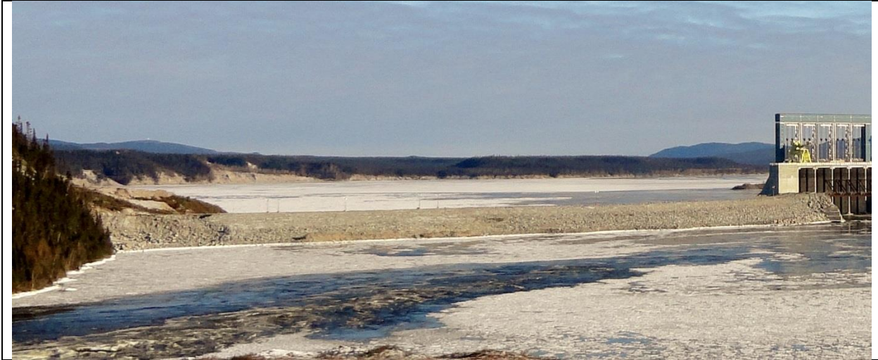
Photo D.1: Upstream face of the cofferdam. (November 30, 2016)
