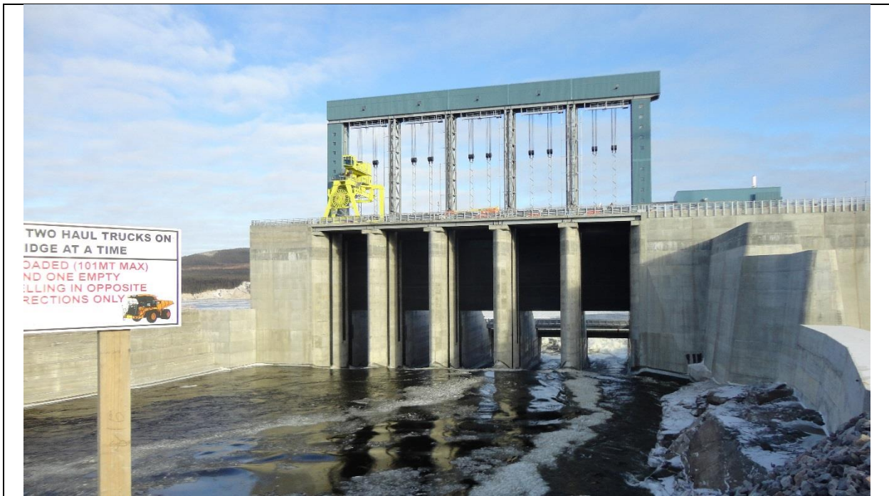
Photo C.2: Spillway – upstream approach channel. (November 30, 2016)
