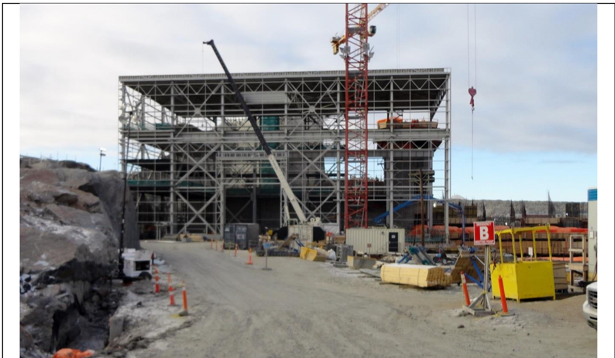
Photo B.8: Structural steel framework erected at South Service Bay. (November 30, 2016)
