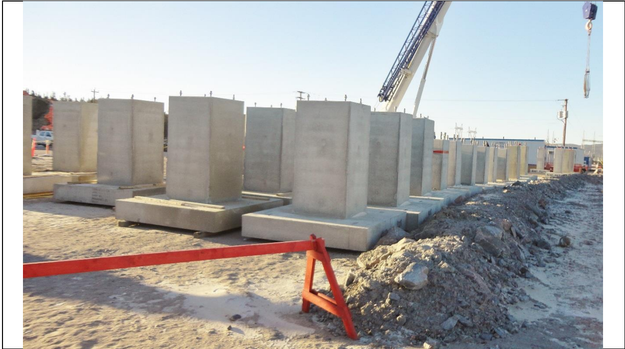
Photo F.5: Prefabricated concrete footings for switchyard equipment foundations. (November 30, 2016)
