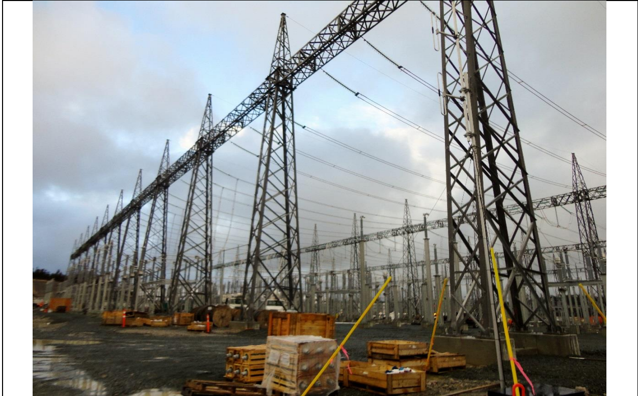
Photo A.1: AC switchyard. (November 29, 2016)
