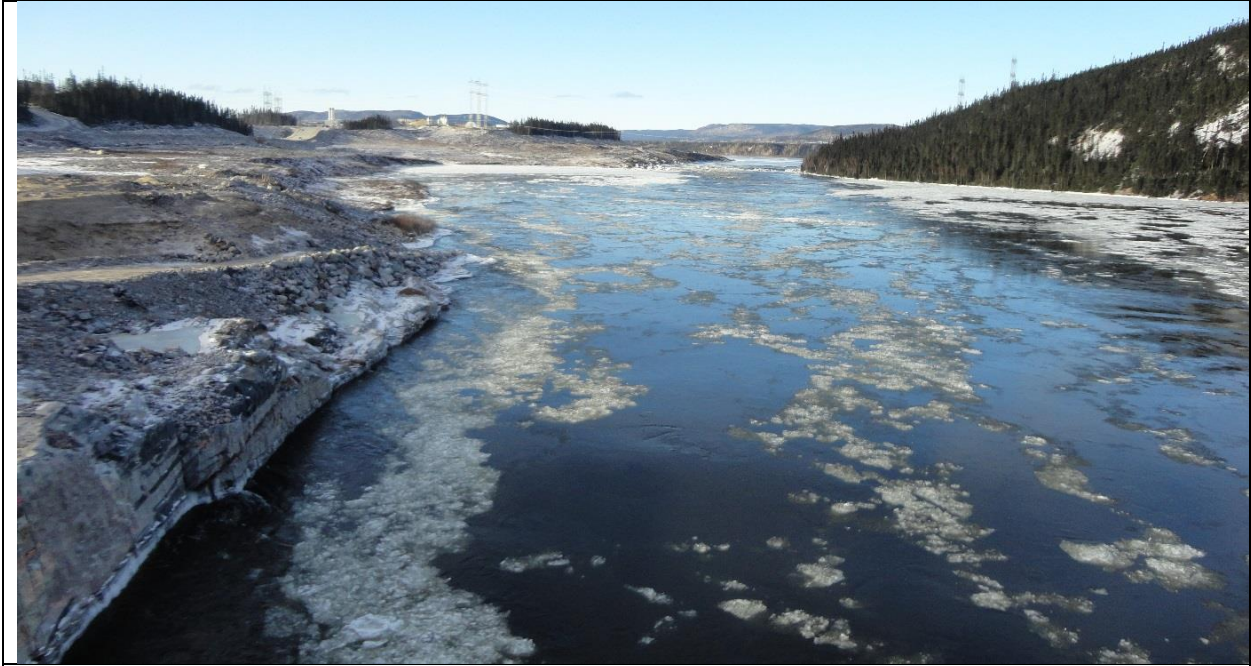
Photo C.5: Spillway intake channel looking upstream from the deck of the temporary bridge.
