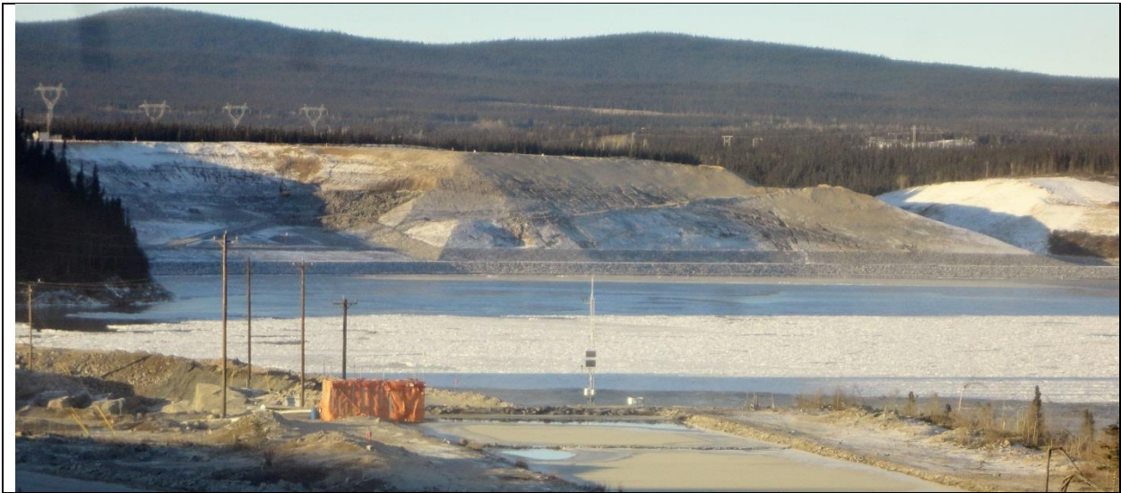
Photo E.2: Downstream face of the North Spur. (November 30, 2016)
