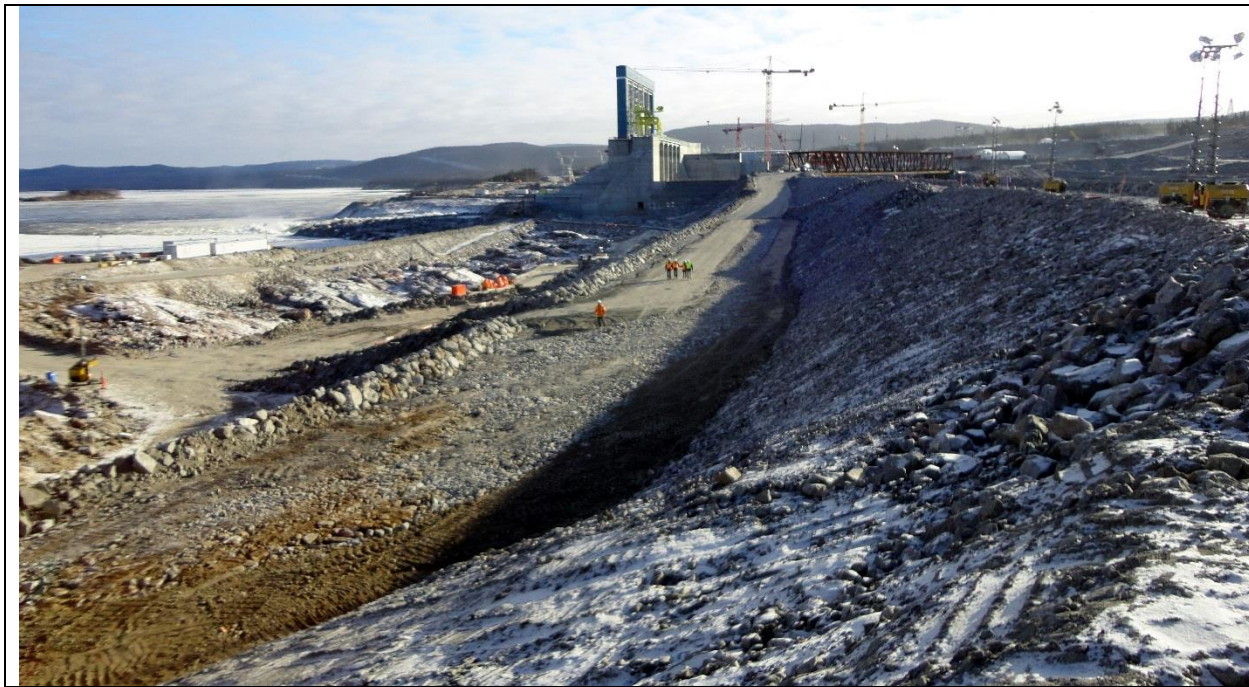
Photo D.6: Downstream el 19 berm, looking south. (November 30, 2016)
