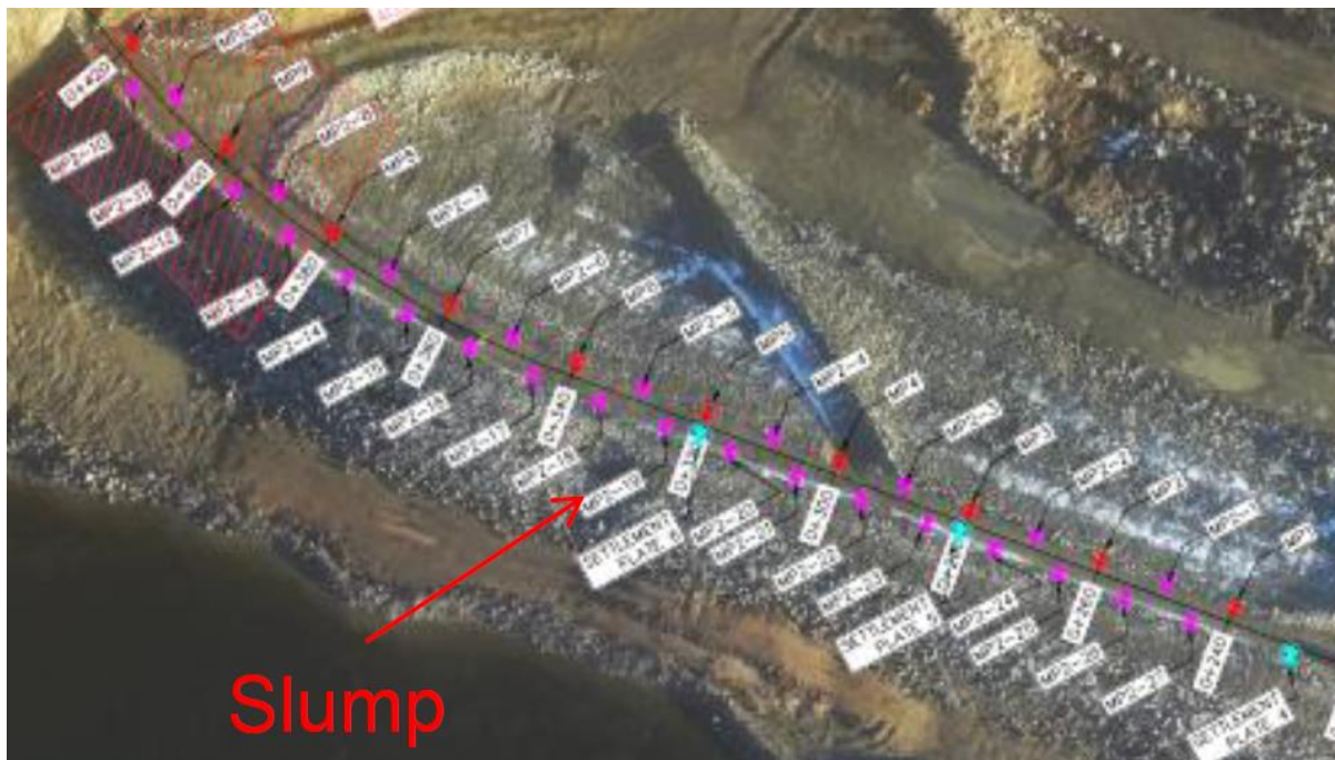
Figure 5.2: Aerial view of cofferdam showing location of the upstream slope slump at approximate Sta 0+330.
