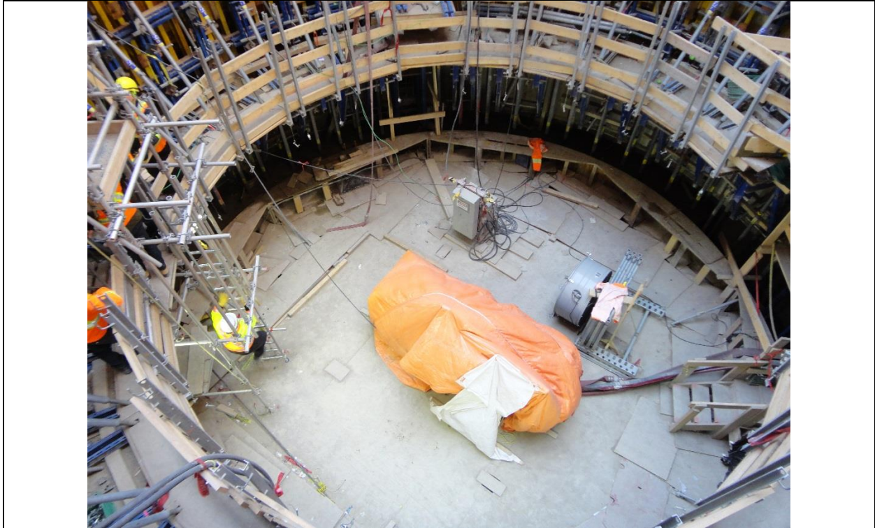
Photo B.7: Unit 2 formwork construction. (November 30, 2016)
