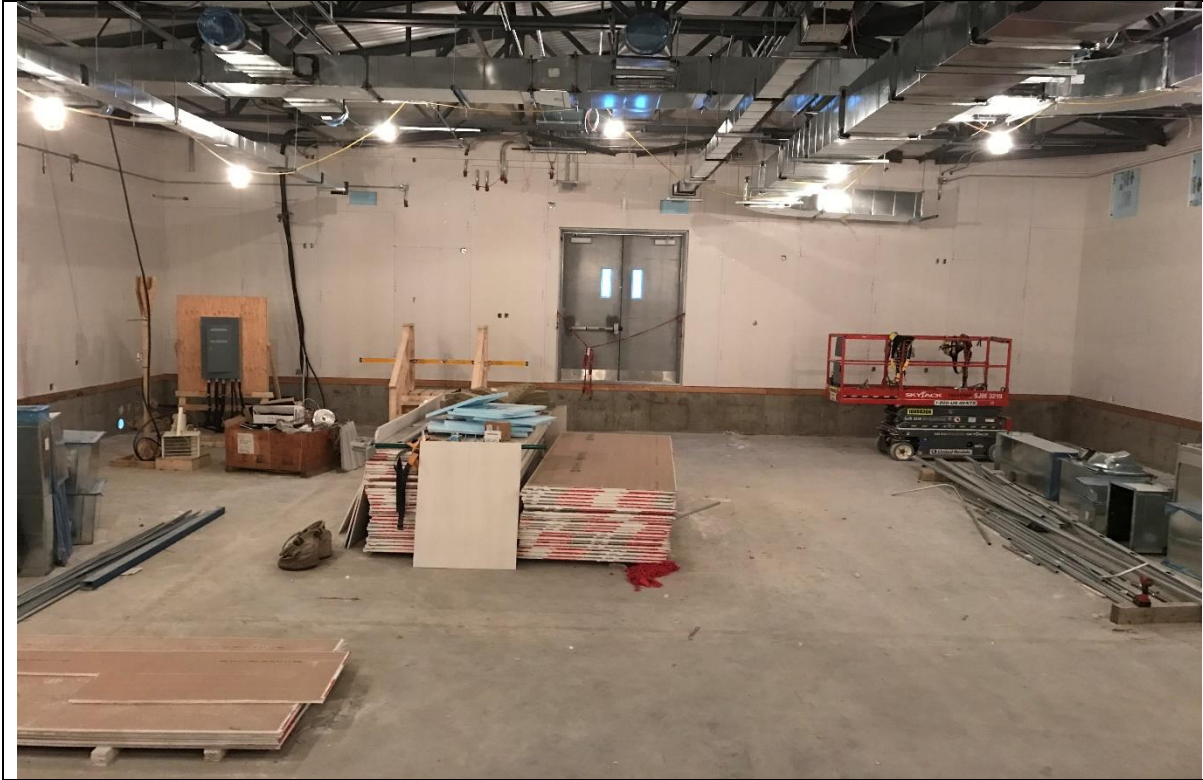
Photo F.11: .AC switchyard control building – interior BOP work underway. (November 30, 2016)
