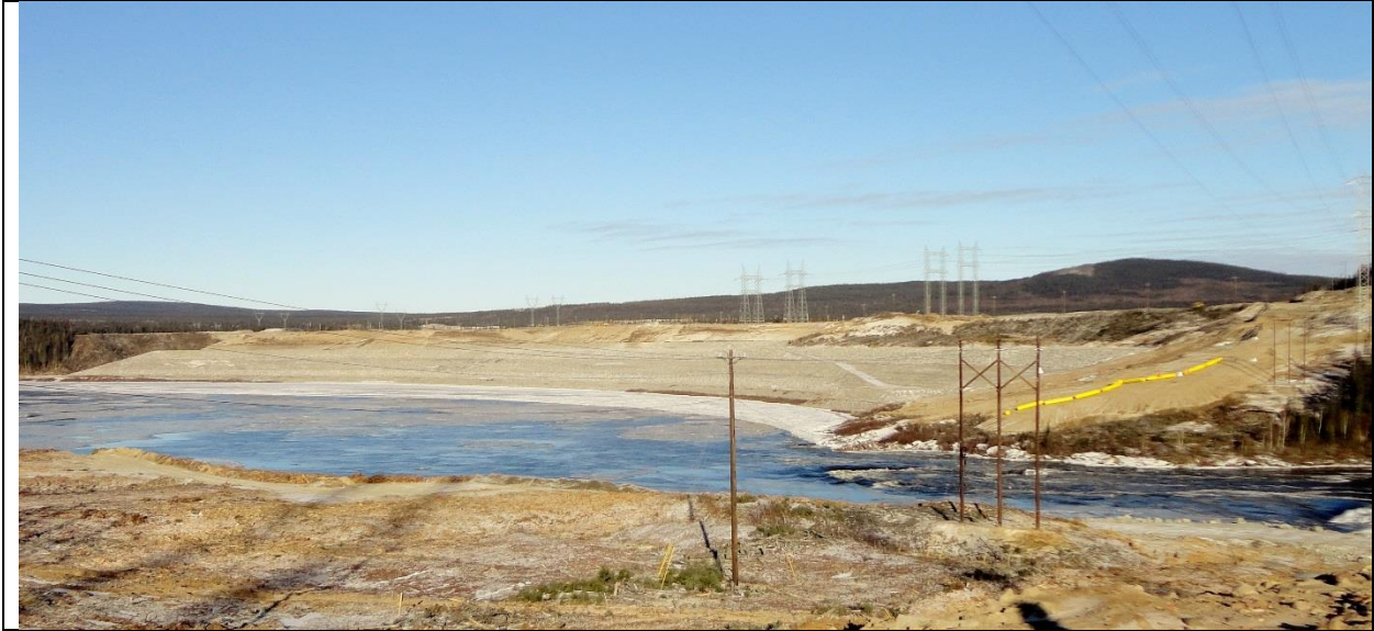
Photo E.1: Upstream face of the North Spur. (November 30, 2016)
