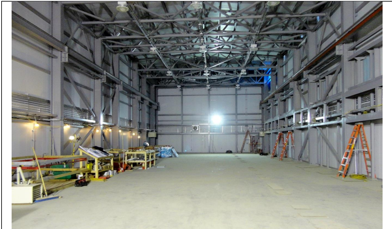
Photo F.10: Interior view of the GIS building. (November 30, 2016)
