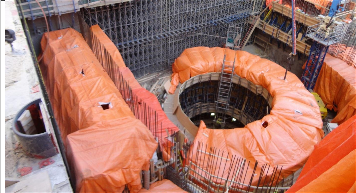
Photo B.11: Unit 1 formwork and weather protection hoarding. (November 30, 2016)
