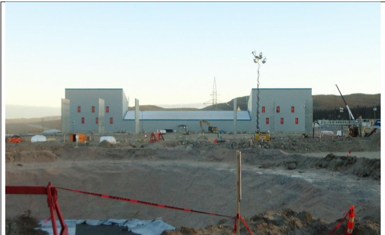
Photo F.2: AC/DC Converter Building, view from the north. (November 30, 2016)
