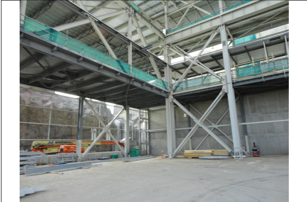
Photo B.9: Interior of the South Service Bay. (November 30, 2016)
