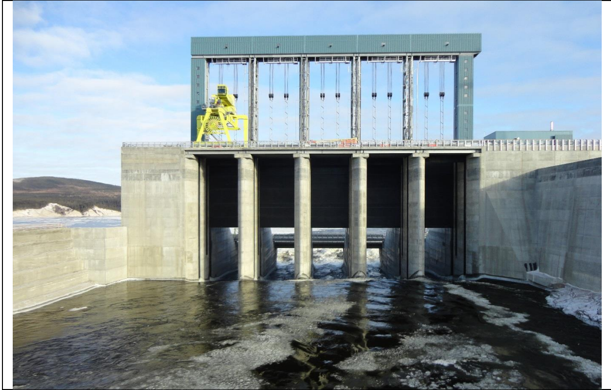
Photo C.1: Upstream view of Spillway. (November 30, 2016)
