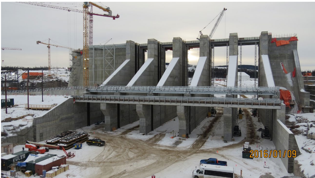
Progress on the Spillway at the Muskrat Falls Site – January 2016
