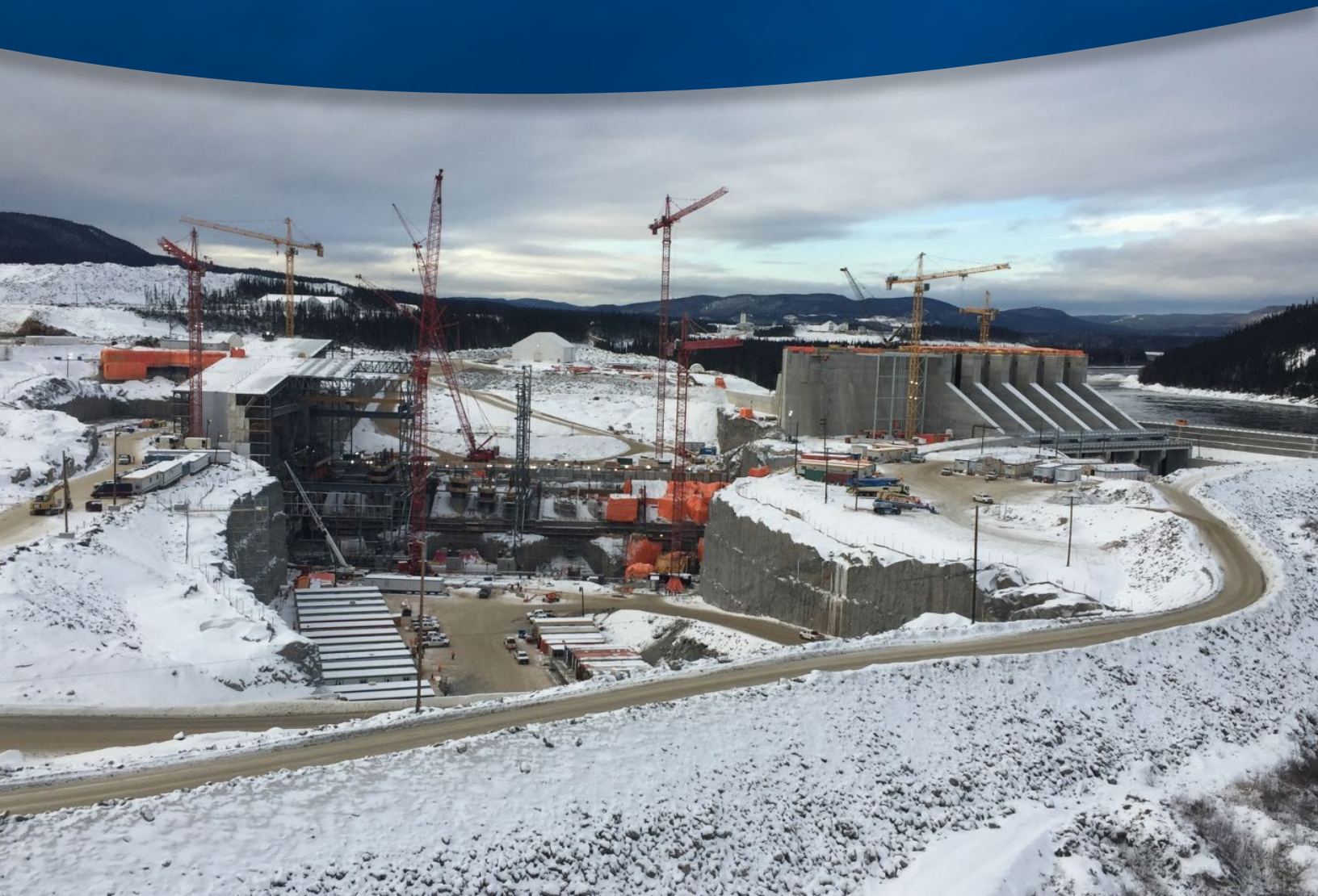
Muskrat Falls Site – Progress on Spillway and Powerhouse – December 2015
