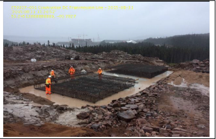
CT0319: Construction of HVac Transmission Line-L2-7
