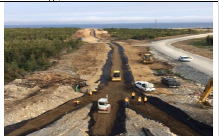
SOBI: Sand installation in cable trenches at Shoal Cove
