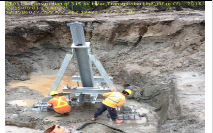
CT0319: Construction of HVac Transmission Line-Rock grillage assembly at L1-290
