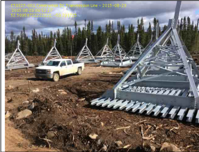
CT0327-001: HVdc Transmission Line—Assembled steel grillages
