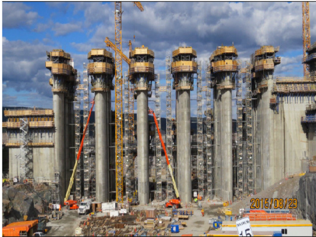
CH0007: Spillway-as seen from Cofferdam 1
