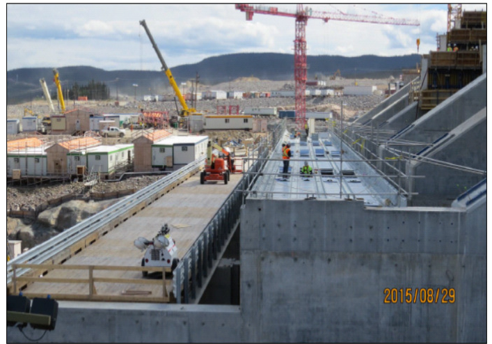
CH0007: Downstream temporary/permanent spillway bridges
