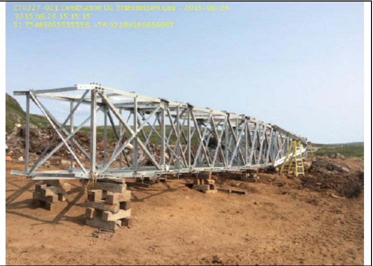
CT0327-001: HVdc Transmission Line—Tower assembly
