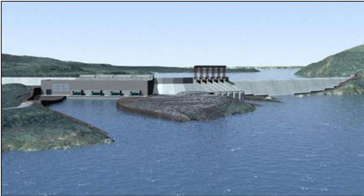
Figure 6-1 Muskrat Falls Generating Facility
