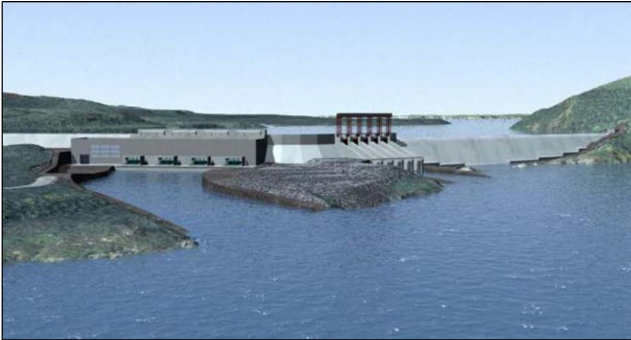
Figure 6-1 Muskrat Falls Generating Facility
