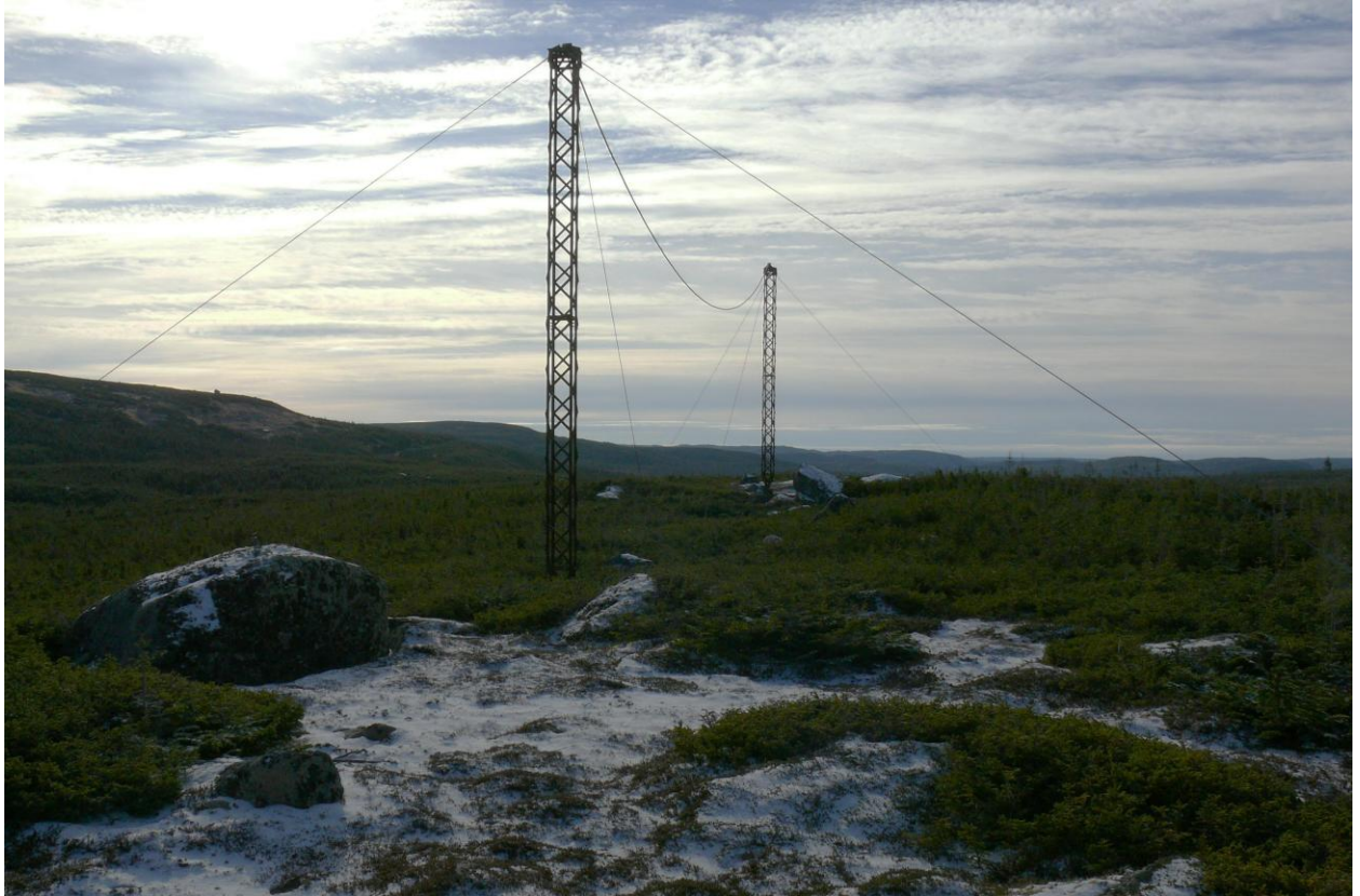
Figure 3: NLH Test Span in the Long Range Mountains, as photographed in 2010
