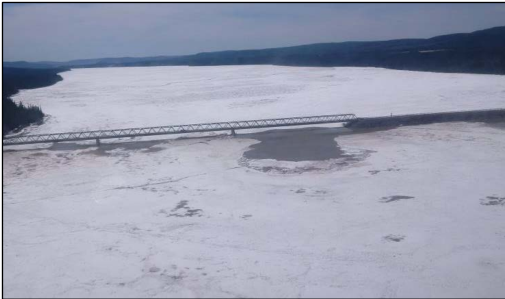
Figure 4-17: Looking Upstream Towards Memorial Bridge (23 km)
