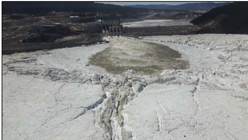
Figure 4-21: Looking Upstream Towards Muskrat Falls (42 km)
