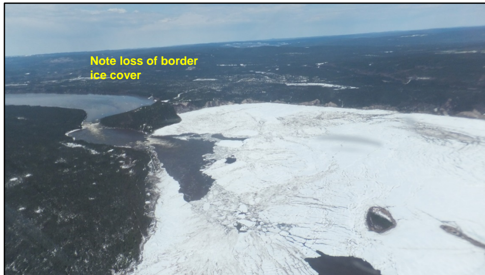
Figure 3-6: May 15, 2012 – Photo Looking Upstream at Muskrat Falls
