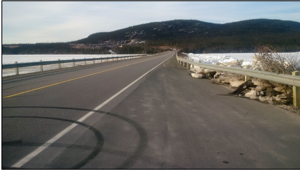
Figure 4-18: Looking Across Veteran Memorial Bridge on May 15
