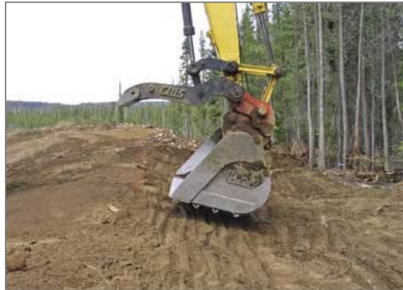
Figure 5-21: Photograph of grooving slope treatment method
