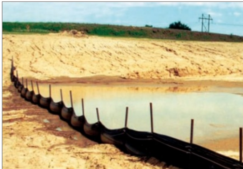
Figure 5-33: A well constructed silt fence
