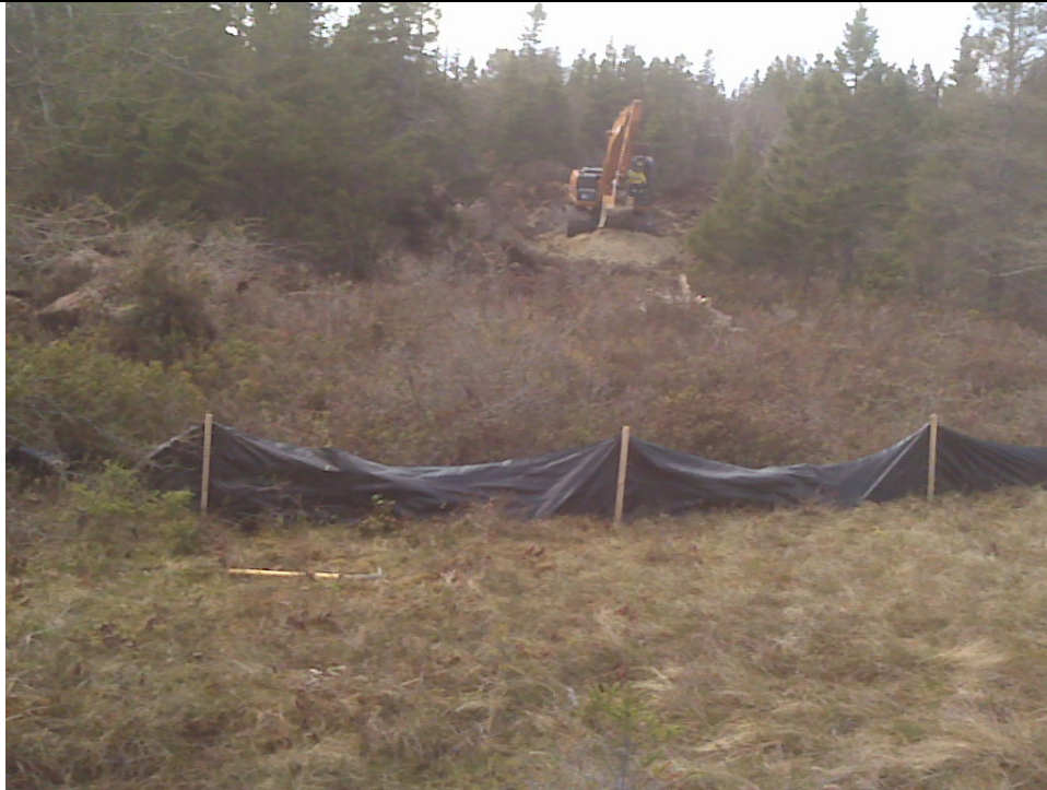
Photo 1: Synchronous condenser trench in early stages of excavation.
