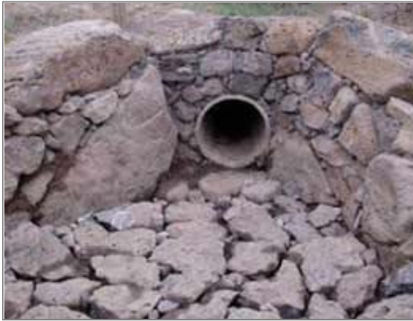
Figure 5-31: Correct Construction of Rock Energy Dissipaters
