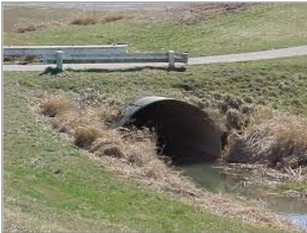
Figure 5-7: Example of well installed culvert
