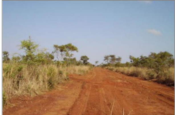
Figure 5-14: Example of grubbed and cleared path
