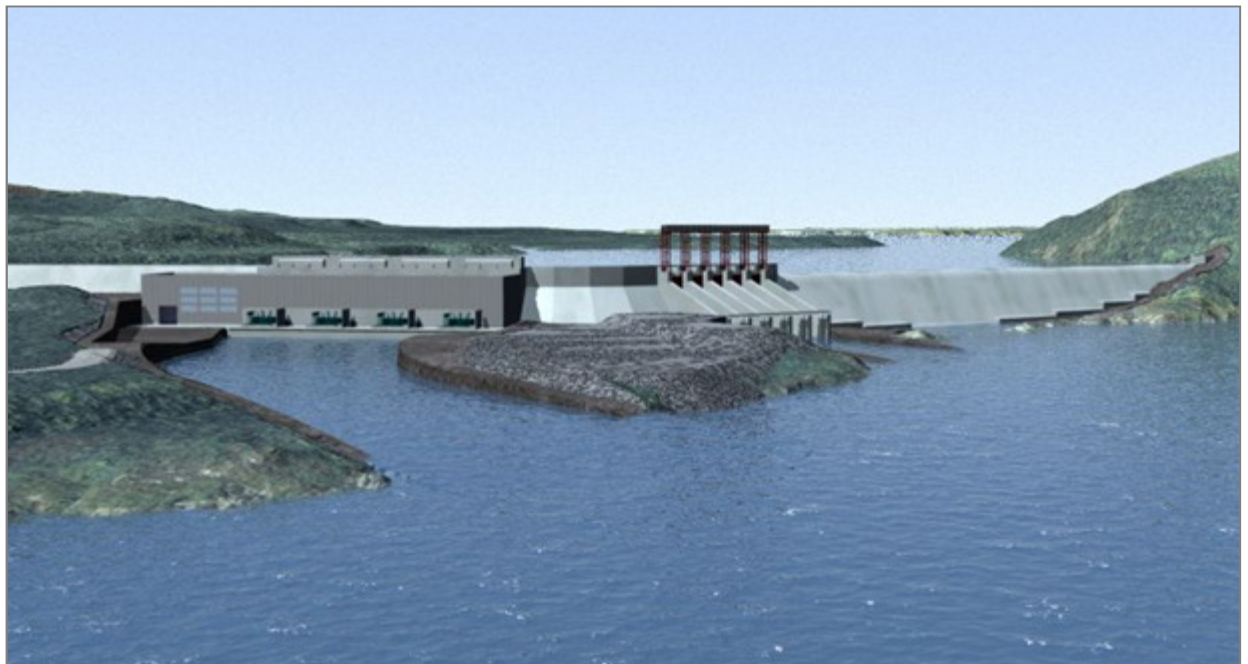
Figure 2-1: Muskrat Falls Generating Facility (Component 1)
