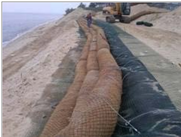
Figure 5-25: Photograph of Fibre Rolls used to stabilize
