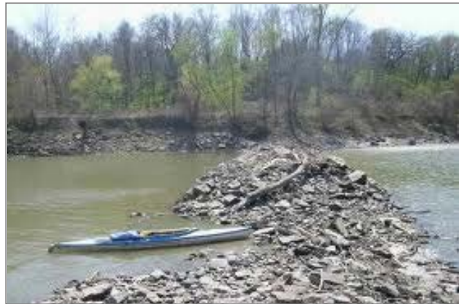
Figure 5-30: Photograph of a Rock Constructed Dike
