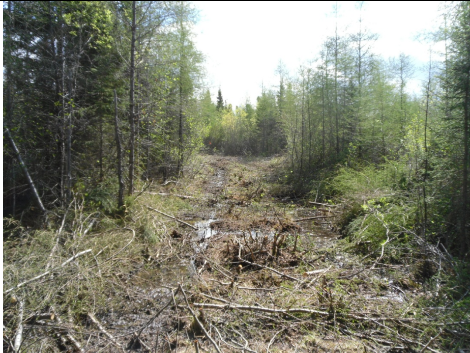
Photo 5: Typical ground conditions.
