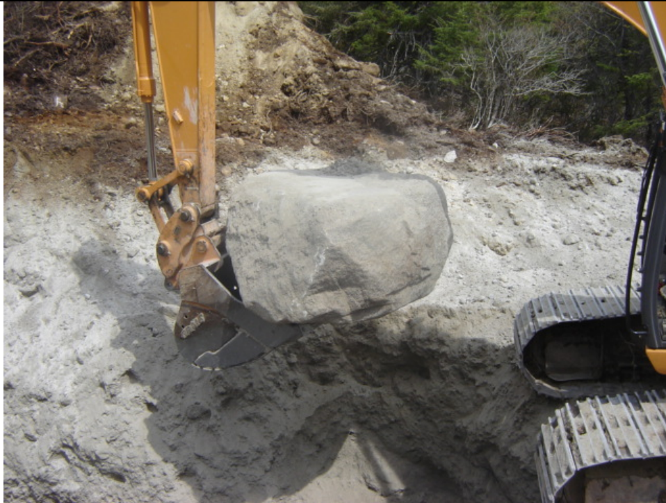
Photo 3: Large boulder excavated from trench.
