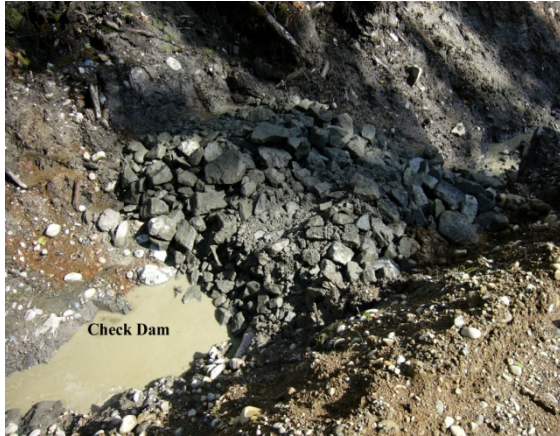
Figure 5-29: Photograph of Rock Constructed Check Dam
