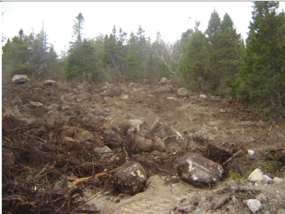
Photo 6: Trench upon completion.
