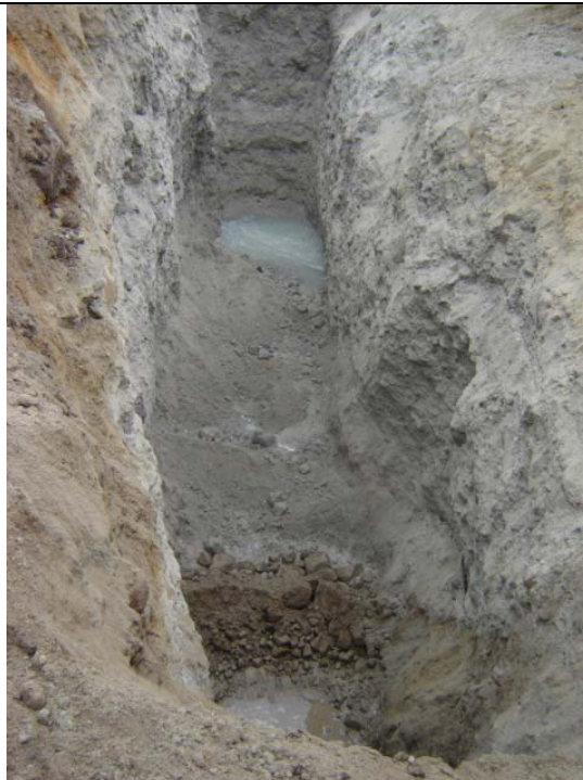
Photo 4: Ground conditions at the west end of the trench.
