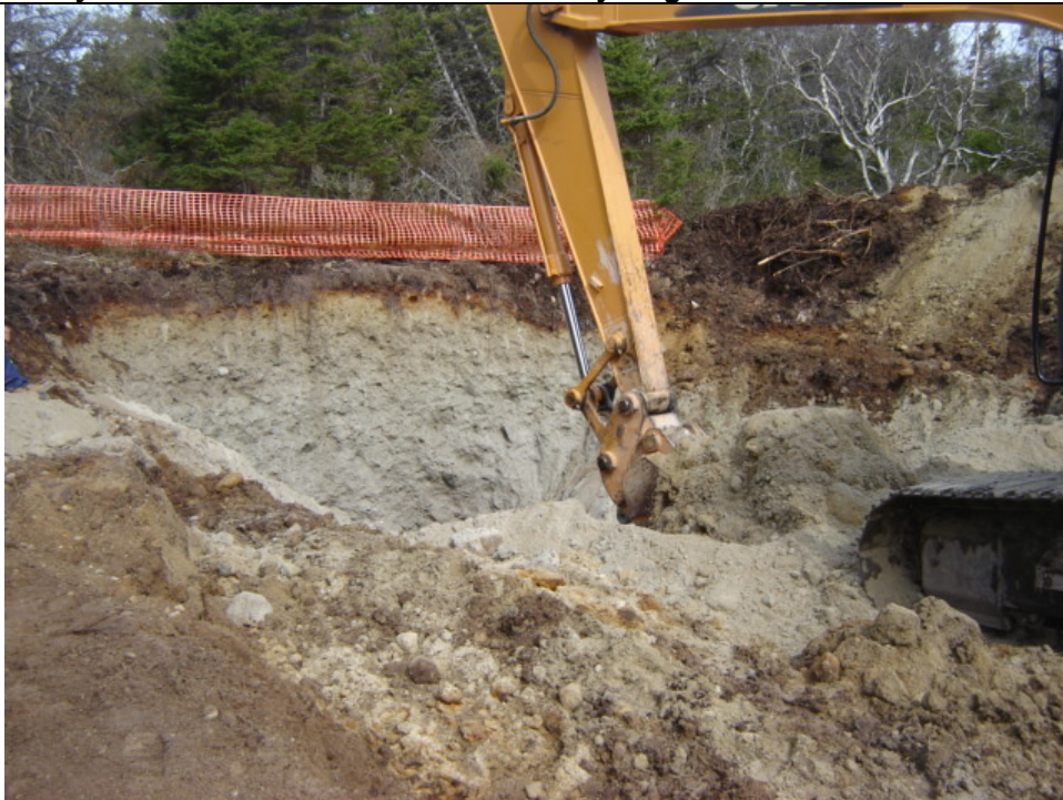
Photo 2: Till excavated from trench.
