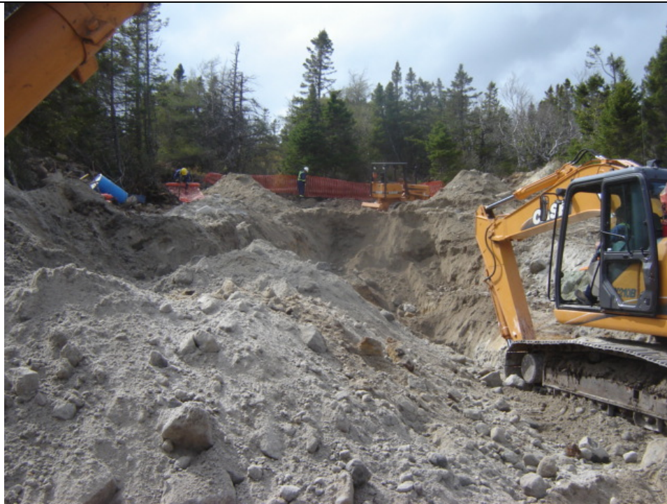
Photo 5: Till excavated from the trench.
