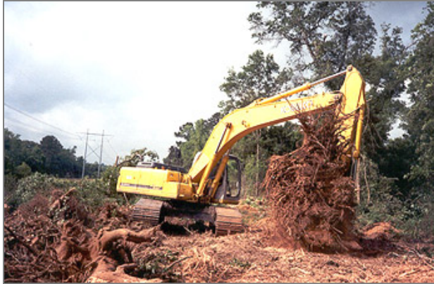
Figure 5-13: Example of grubbing activities
