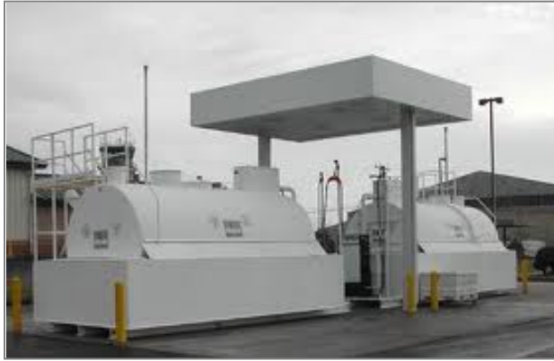
Figure 5-5: Acceptable fuel storage with dykes
