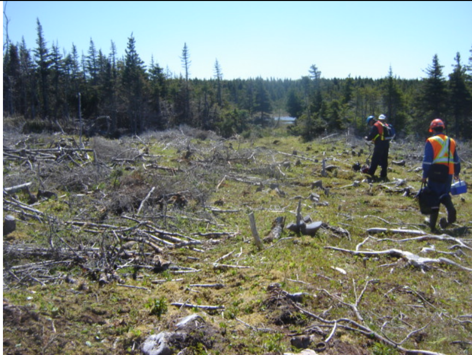
Photo 9: Typical site conditions.
