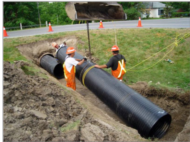
Figure 5-8: Example of culvert installation
